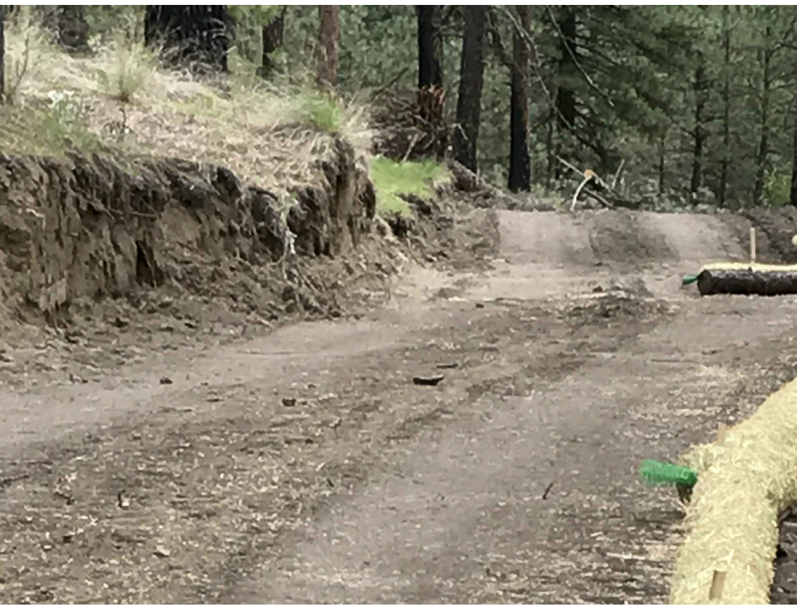
4. HIGH ROAD CUT/FILL
