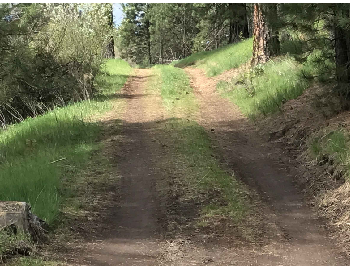
1. EXISTING ROAD CONDITIONS
