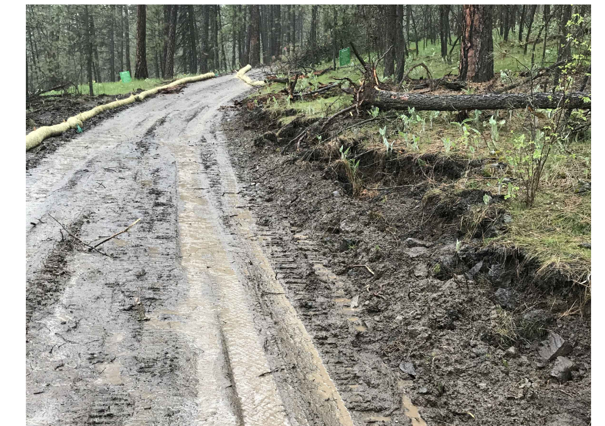
8. MODERATE ROAD CUT/FILL
