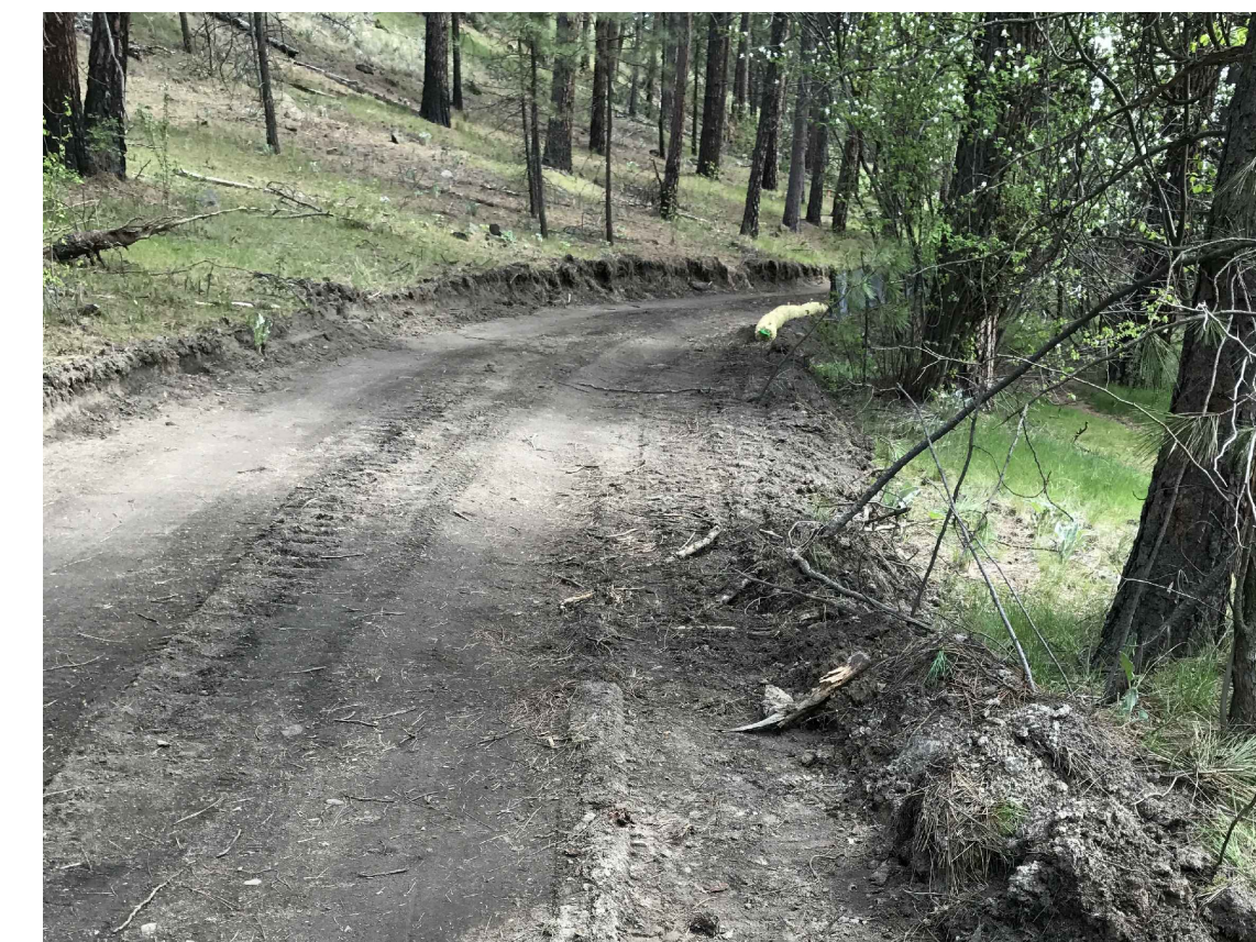
3. MODERATE ROAD CUT/FILL
