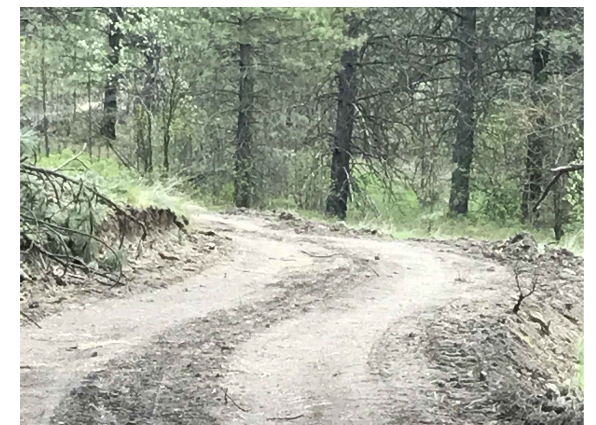
5. MODERATE ROAD CUT/FILL
