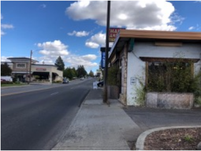
Figure 5: Encroachment on sidewalk of utility pole.
