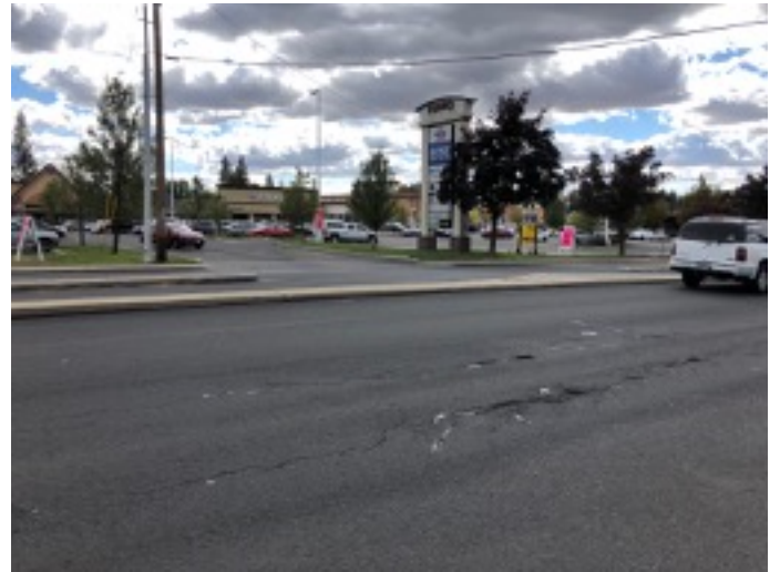
Figure 9: Blocked intersection at Hatch Street.
