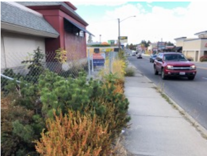
Figure 6: Vegetation and fencing encroaching on sidewalk.
