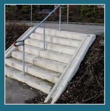
STAIR WITH BIKE RUNNEL Stairs within South Hill's pedestrian network should be designed with features that facilitate easier bicycle handling. A bike runnel is a track on a staircase that allows you to roll your bicycle up with you as you walk.
