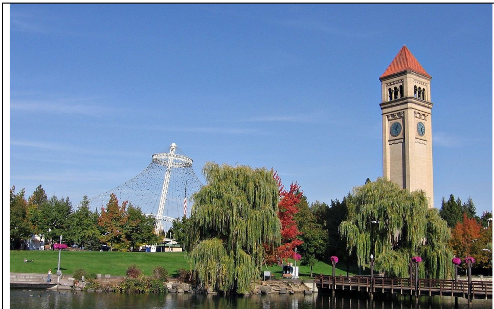
Great Northern Railway Depot Clock Tower at Spokane's Riverfront Park.
