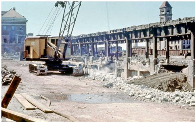
View of demolition of elevated trestles in railyard area as part of preparations for Expo '74.
