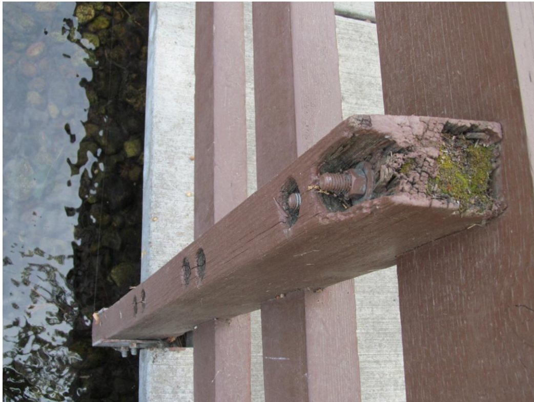
Photo 7 – Rotted Timber Railing Post
