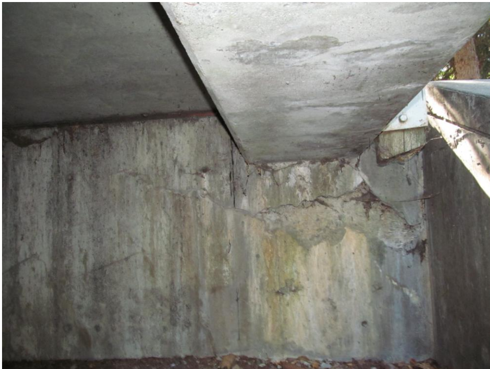
Photo 8 – Spall in Abutment Backwall
