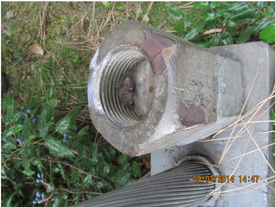
Photo 12 – Lock Nut at Southwest Anchorage is only 30% Engaged
