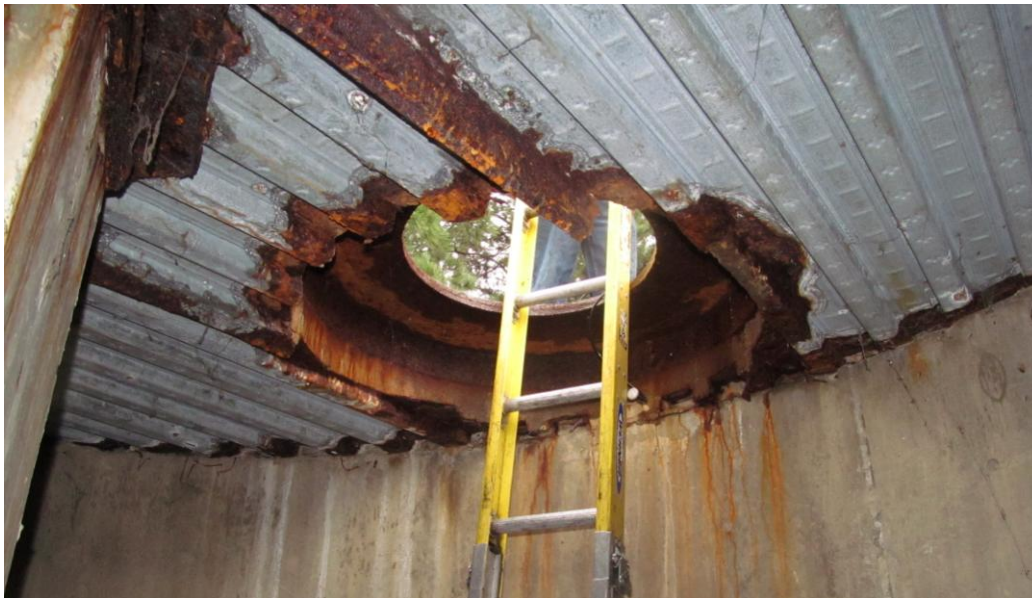
Photo 15 – Corroded Stay-in-Place Formwork around Manhole
