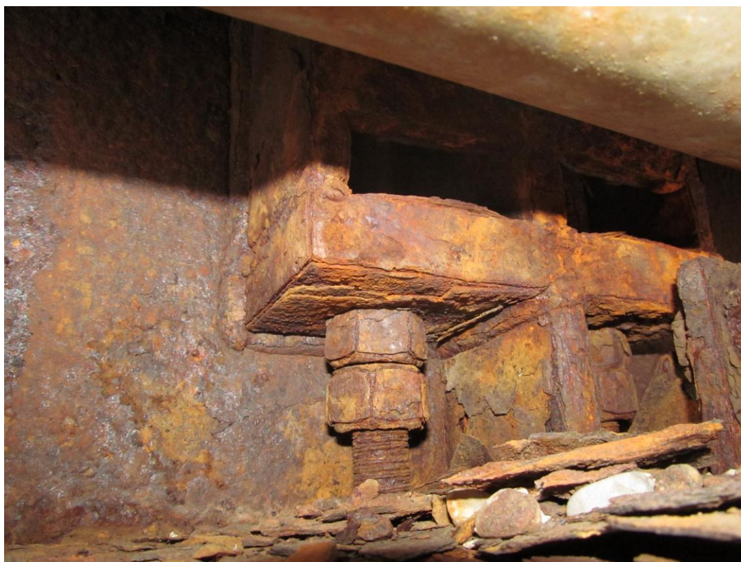
Photo 10 – Moderate to Heavy Corrosion at Interior Suspender Cable Connection (H5 RT)
