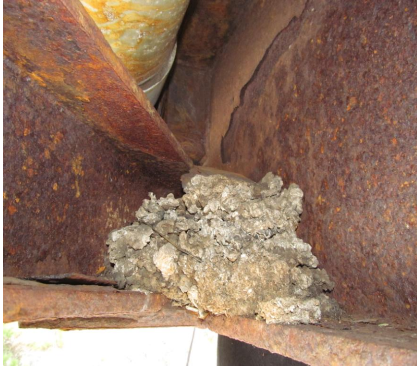
Photo 7 – Debris at Panel Point (Typical)
