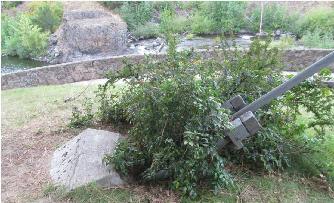
Photo 11 – Shrubs around Cable/Threaded Rod, Partially Buried Concrete Block
