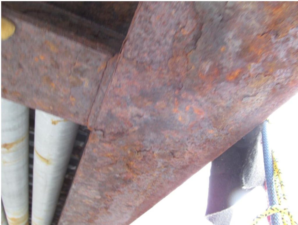
Photo 6 –Moderate Corrosion Bottom Flange of Left Girder at H5
