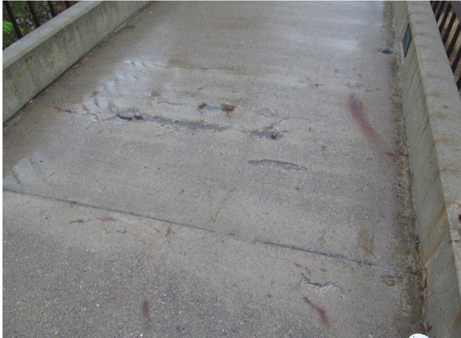
Photo 3 – Exposed Rebar in Deck
