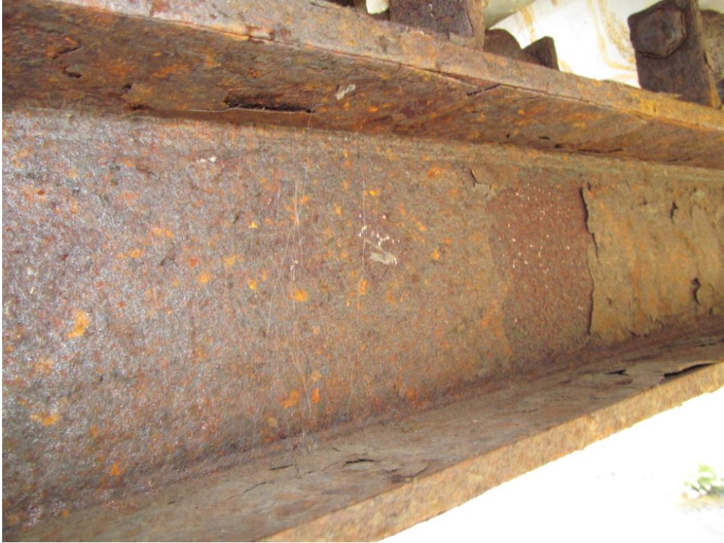
Photo 5 – Moderate Corrosion/Flaking of Floorbeam 1-13
