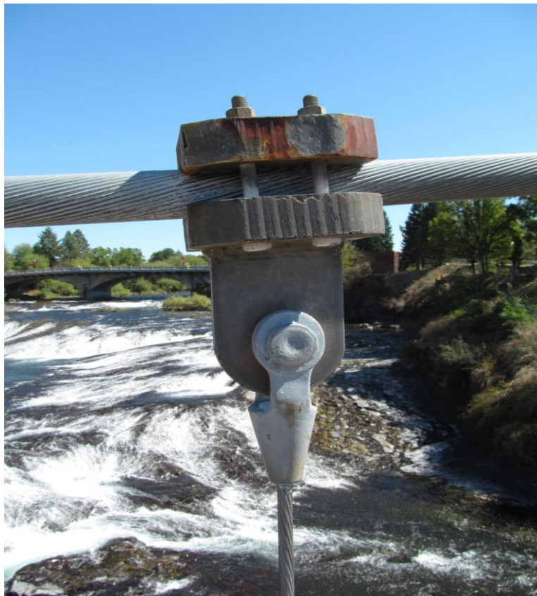
Photo 8 – Typical Suspender Cable Connection
