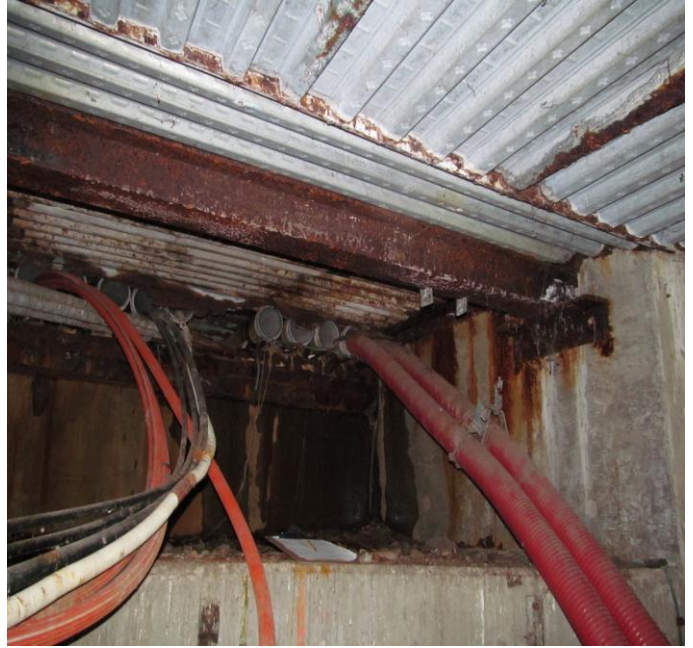
Photo 14 – Corroded/Missing Stay-in-Place Formwork and Corroded Beam/Angle in Vault No. 3 near Abutment
