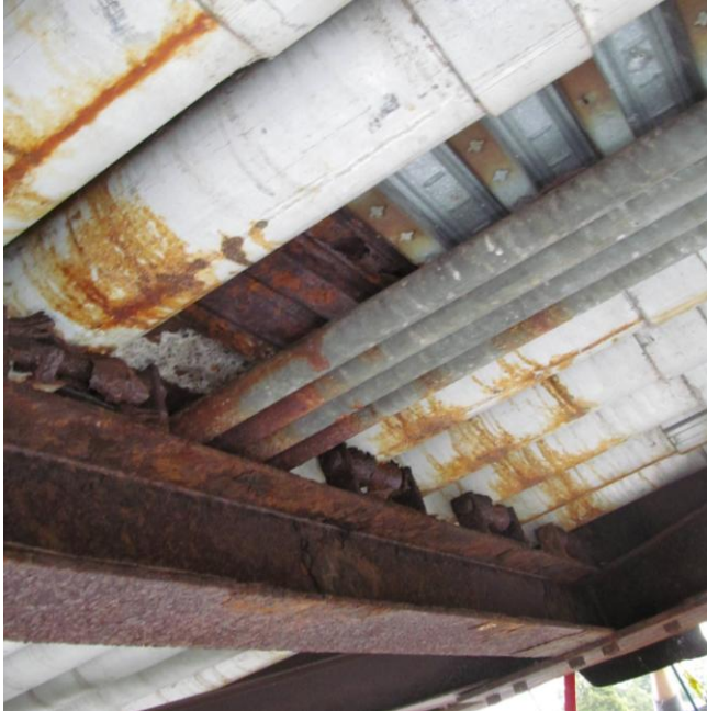
Photo 13 – Corroded/Missing Stay-in-Place Formwork above Floorbeam (Typical)
