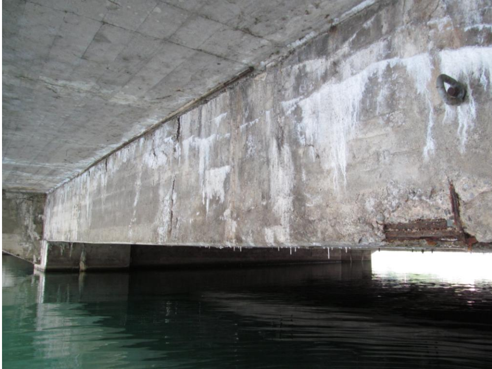
Photo 5 – Typical Condition of Girders – Horizontal Leaching Cracks
