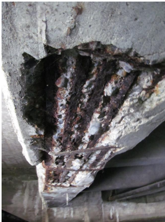
Photo 4 – Typical Condition of Exterior Girders – Exposed/Corroded Reinforcement
