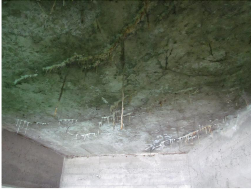
Photo 3 – Typical Soffit Condition - Map Cracking with Efflorescence/Stalactites
