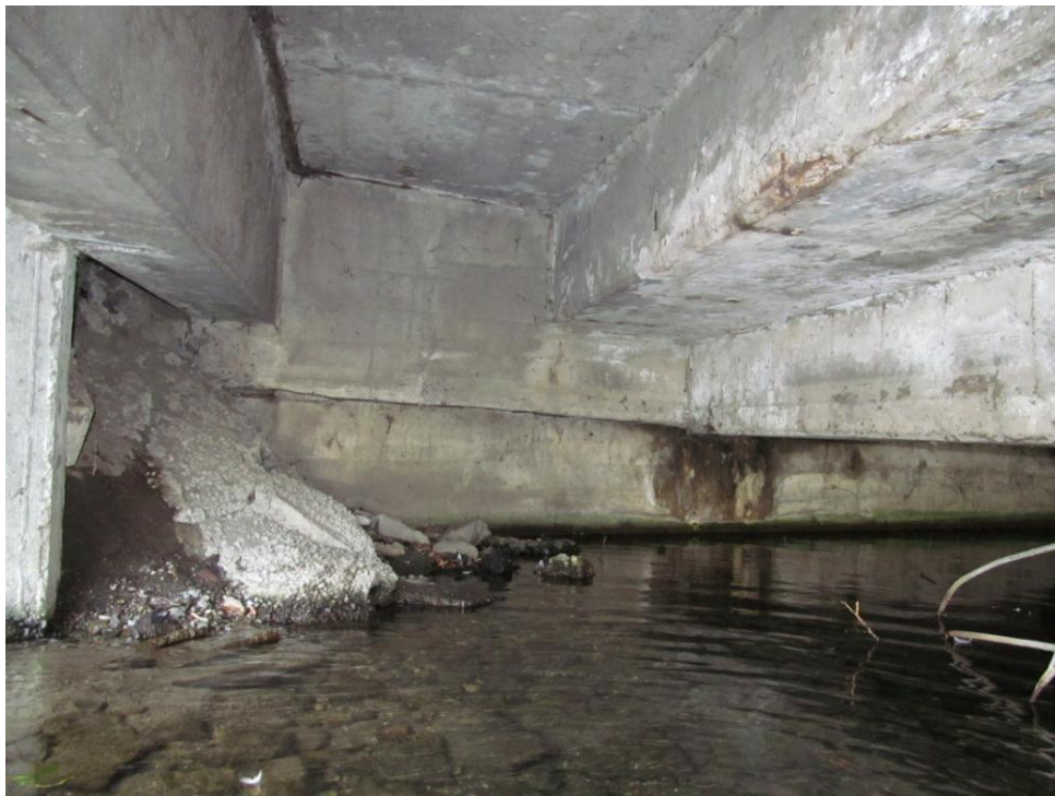
Photo 6 – Material Spilling Through at South Abutment
