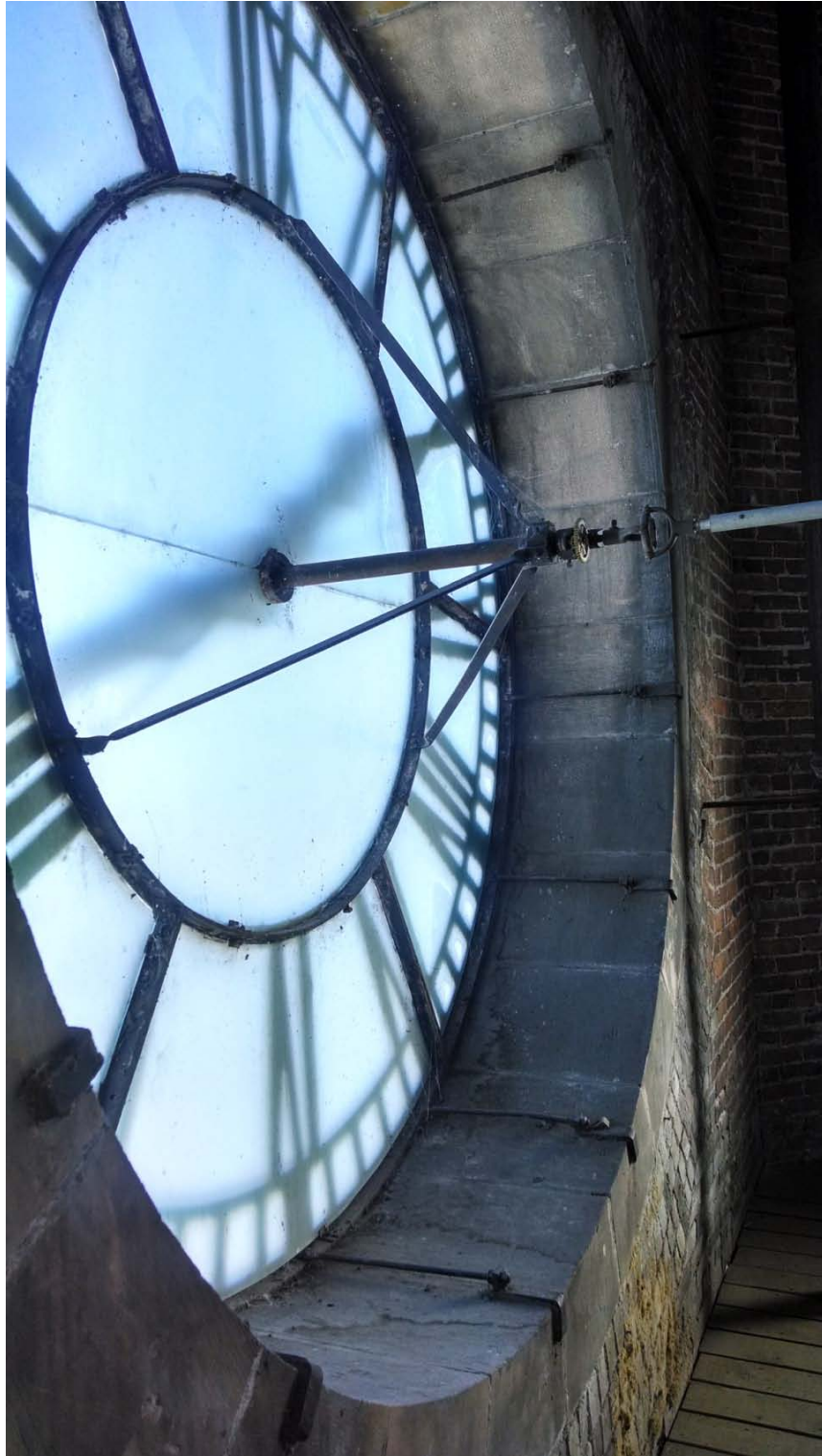
Photo of the Clock Drive Shaft Connection to the Clock Face
