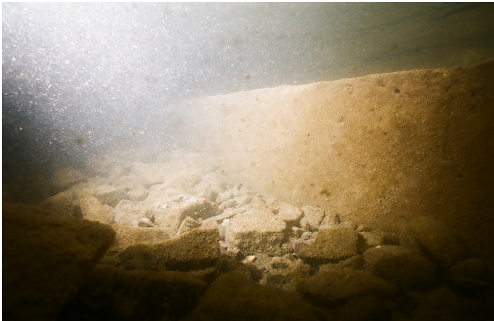
PHOTO No. 10: Abutment No. 9 - Note the good condition of the concrete footing on this abutment. Although no evidence of any undermining was found, the footing was exposed for a height of 4-6 inches along its full length.
