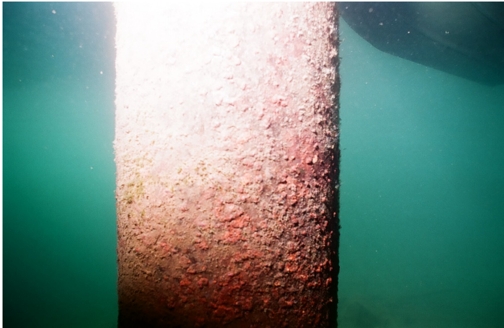
PHOTO No. 5: Bent 4, Row A Pile - Note the general surface corrosion and rust nodules evident on this pile in the submerged zone. This condition was found to be typical of the submerged surfaces of the inspected piling.
