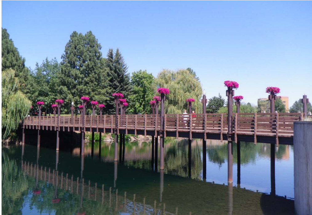
PHOTO No. 1: King Cole Bridge, Looking North - Note the steel girder and beam construction of the superstructure. This bridge is supported on steel pipe piling which extend up above the deck and provide lighting and decorative functions.
