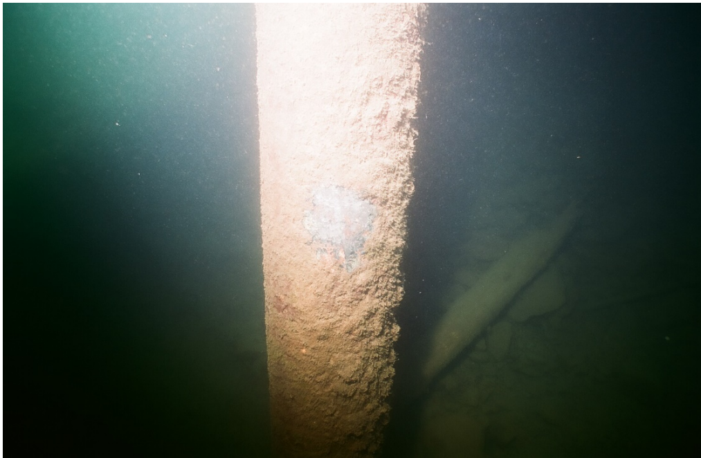
PHOTO No. 7: Bent 7, Row B Pile - Note the generally smooth condition of the steel in the cleaned area. Level II cleaning and Level III ultrasonic thickness readings were taken at this location approximately 6 feet below water. The average steel thickness readings obtained at this location is 0.327 inches.
