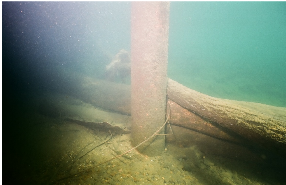
PHOTO No. 6: Bent 4, Row A Pile - Inspection also found general surface corrosion and algae growth evident on this pile at the mudline. This condition was found to be typical of the inspected piling near the channel bottom. Also note the logs that have collected on the upstream side of the bent.
