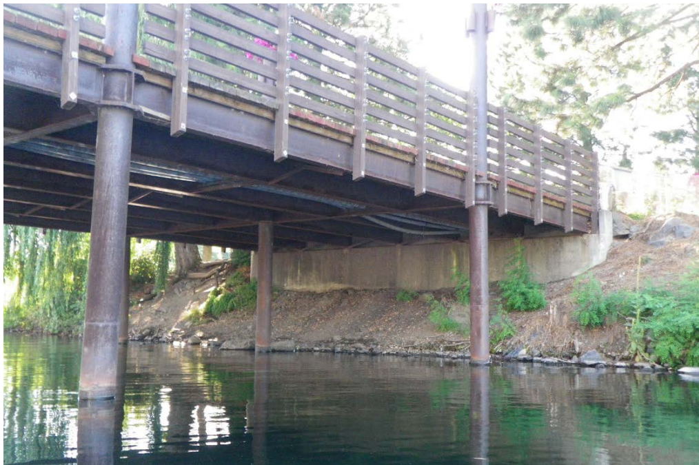
PHOTO No. 2: Abutment No. 1, Looking Northwest - Note the good condition of the concrete which was found to be sound. Also note the general good condition of the steel with minor surface corrosion and the apparent stable condition of the bank.
