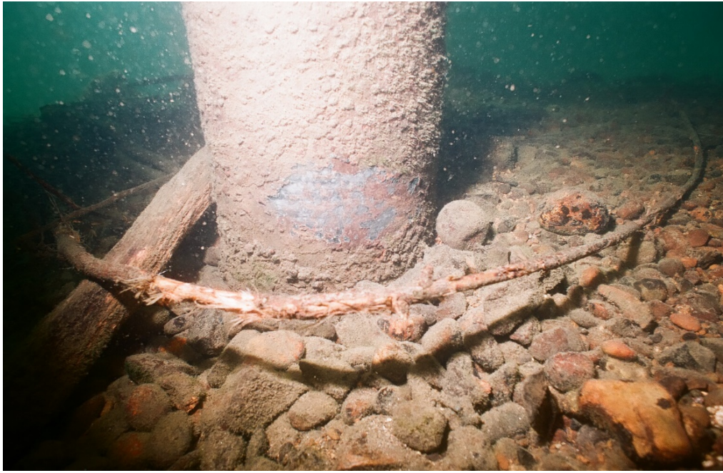
PHOTO No. 9: Bent 4, Row C Pile - This pile was also subjected to Level II cleaning and Level III thickness readings at the mudline. The average steel thickness obtained at this location was 0.392 inches at the mudline. Note the gravel / rock and timber debris evident on the channel bottom.
