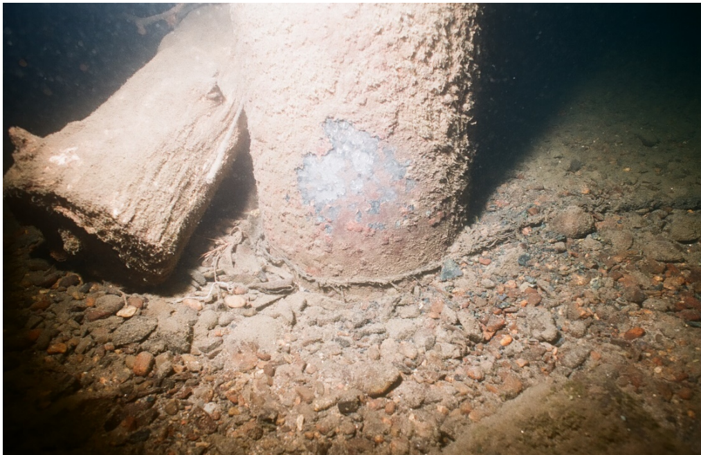
PHOTO No. 8: Bent 7, Row B Pile - This pile was also subjected to Level II cleaning and Level III thickness readings at the mudline. The average steel thickness obtained at this location was 0.345 inches at the mudline. Note the gravel / rock and timber debris evident on the channel bottom.
