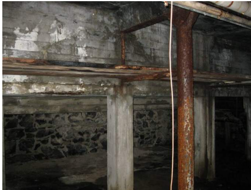
Photo 6: Main Floor Framing at South End (from lower level)
