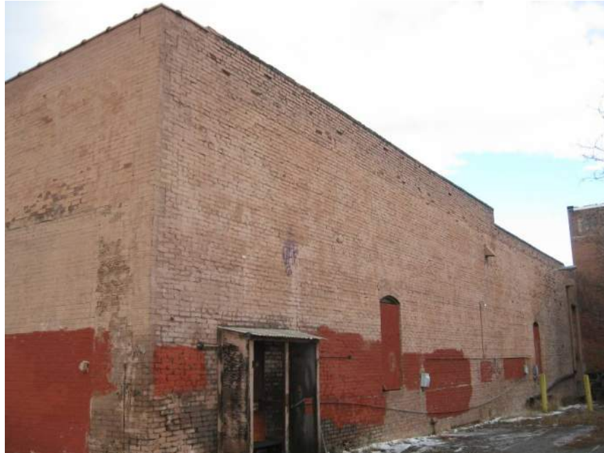
Photo 5: Southeast Corner Exterior Wall
