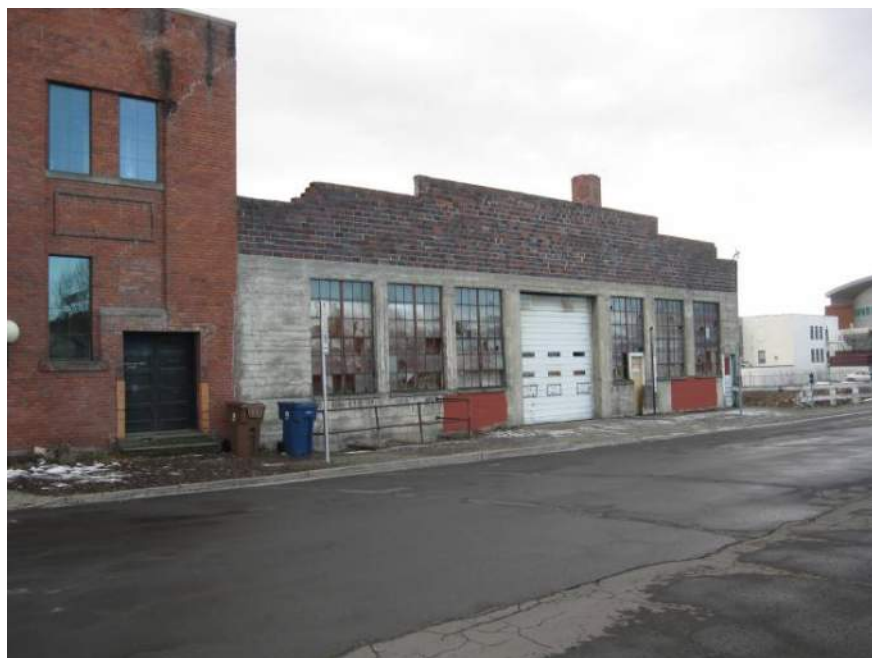
Photo 3: North End Exterior Wall
