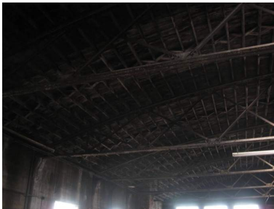
Photo 9: General Roof Framing at North End
