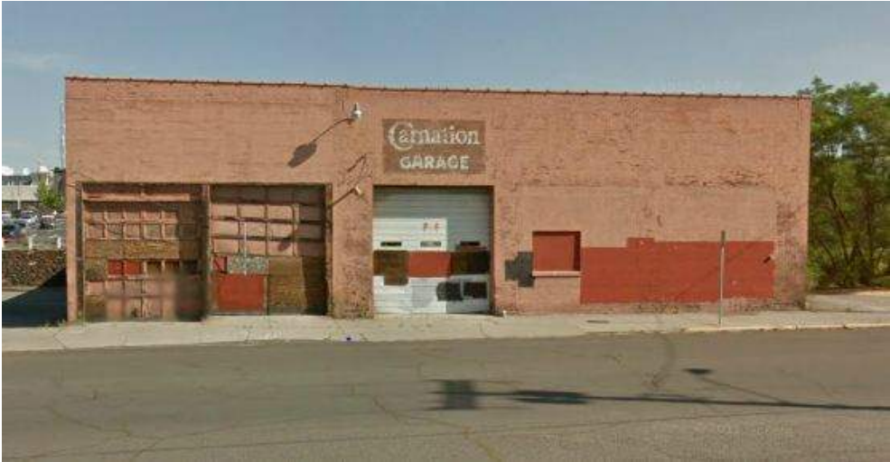
Photo 1: South Exterior Wall Facing Cataldo Avenue
