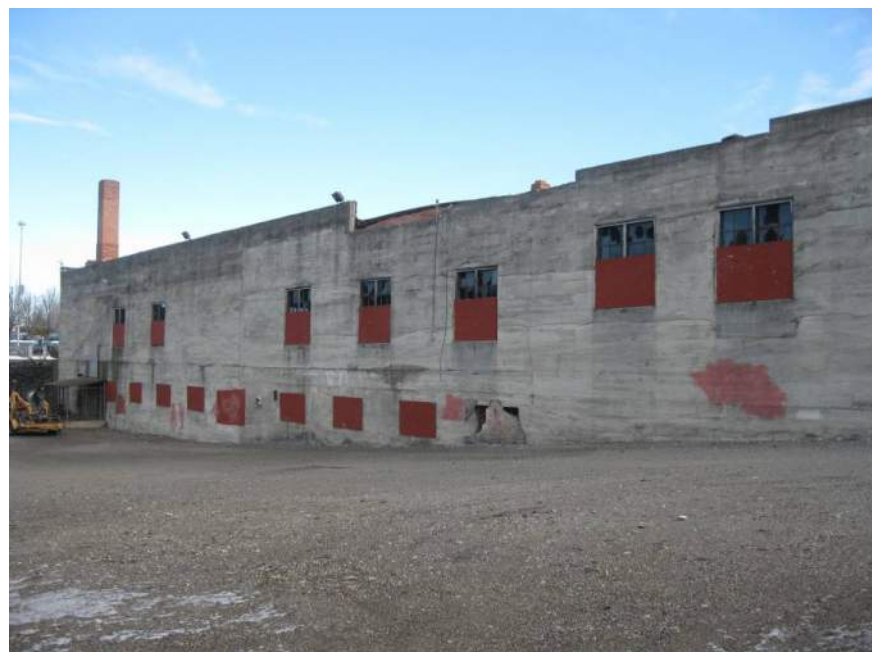
Photo 4: West Side Exterior Wall
