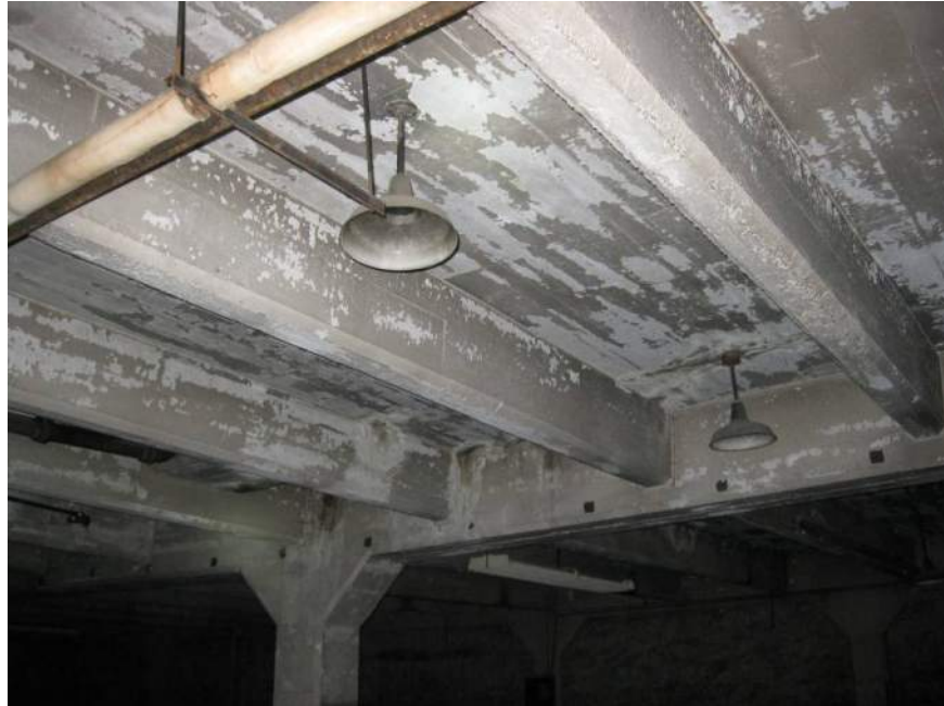
Photo 7: Main Floor Framing at North End (from lower level)
