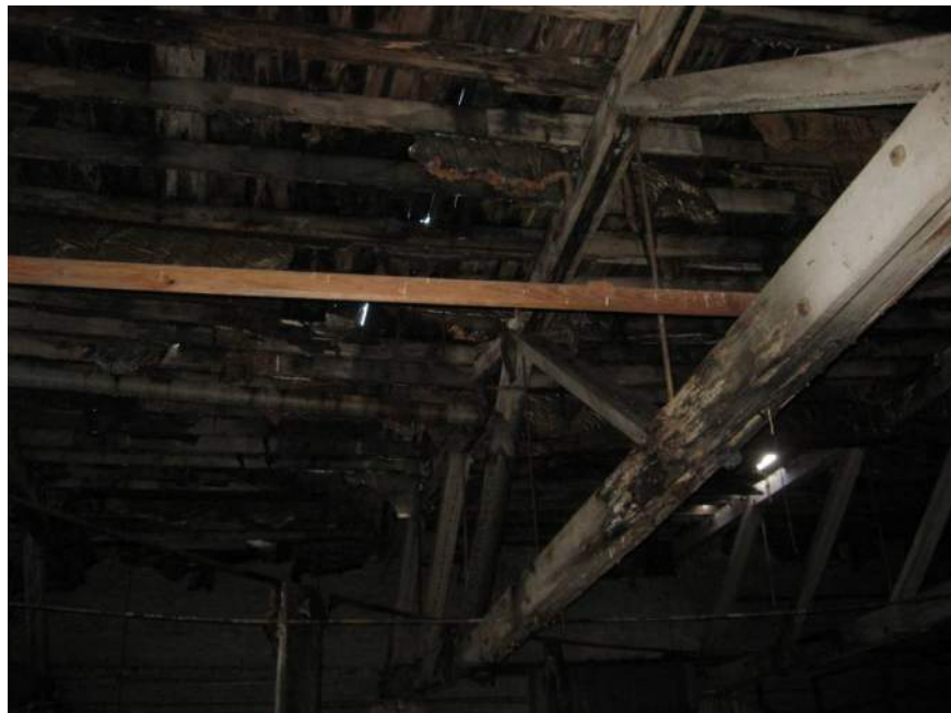
Photo 8: Failed Roof Structure in Southeast Area
