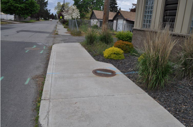
Well 1 Meter Vault
