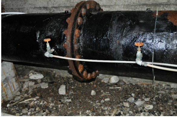
Differential Flow Meter
