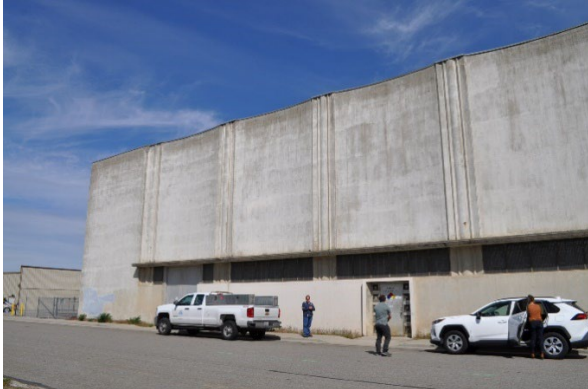
Corner of Building Facing East
