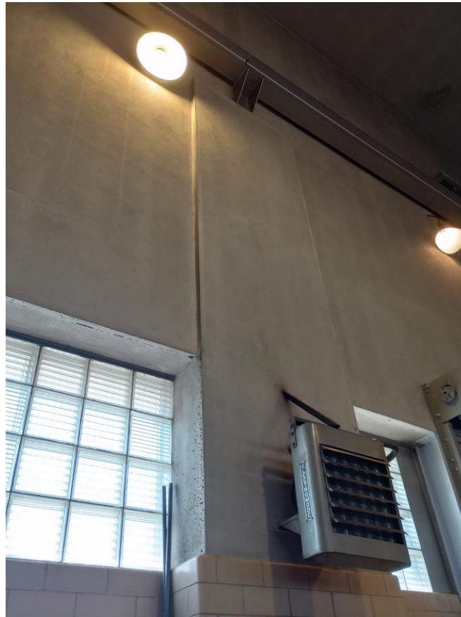
Figure 2-1 | Parkwater – Concrete Walls, Columns, and Ceiling
