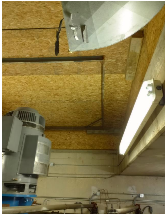
Figure 6-1 | Nevada – Concrete Walls and Timber Ceiling
