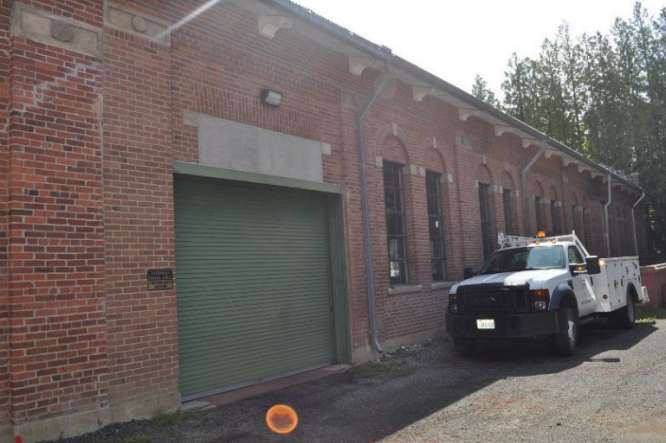
West Exterior of Well Building
