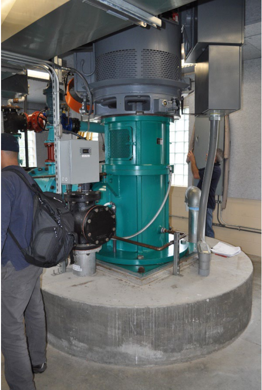
Well 1 Pump Motor
