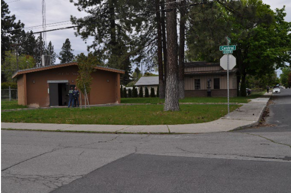
Control Building and Well 2 Building Exterior
