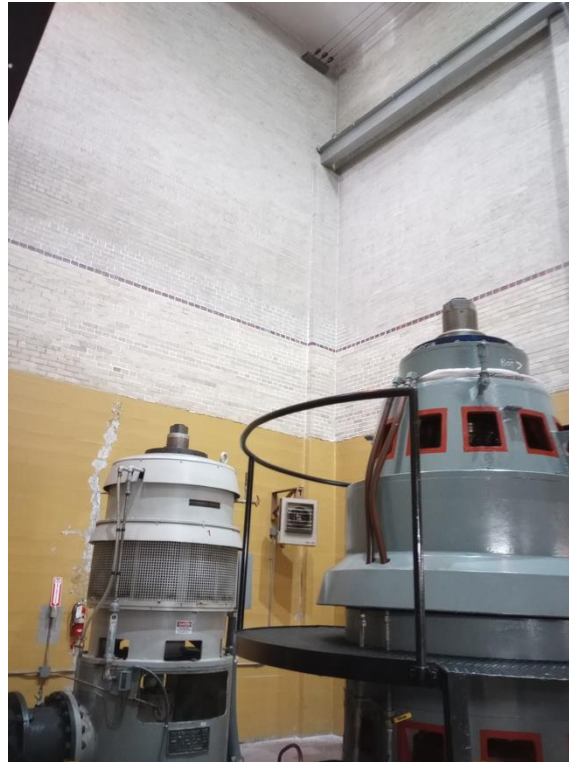
Figure 3-1 | Ray – Unreinforced Masonry Walls and Concrete Foundation (Painted Yellow)
