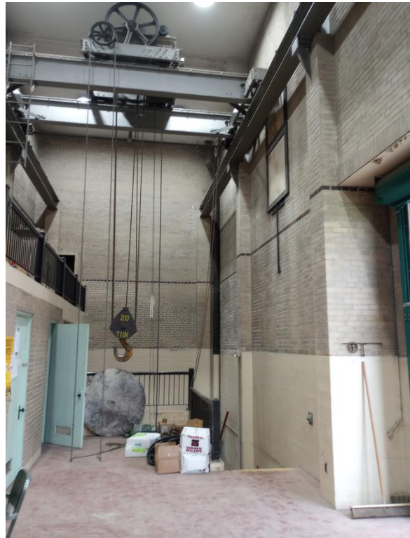
Figure 7-1 | Hoffman – URM Walls on Concrete Foundation and Unknown Ceiling
