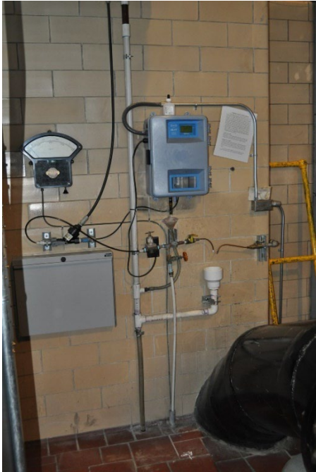
Parkwater Chlorine Monitor
