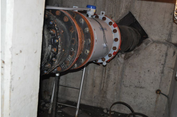
Nevada Flow Meter Tunnel
