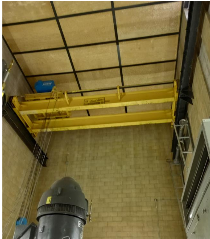
Figure 5-1 | Grace – CMU Walls and Unknown Ceiling
