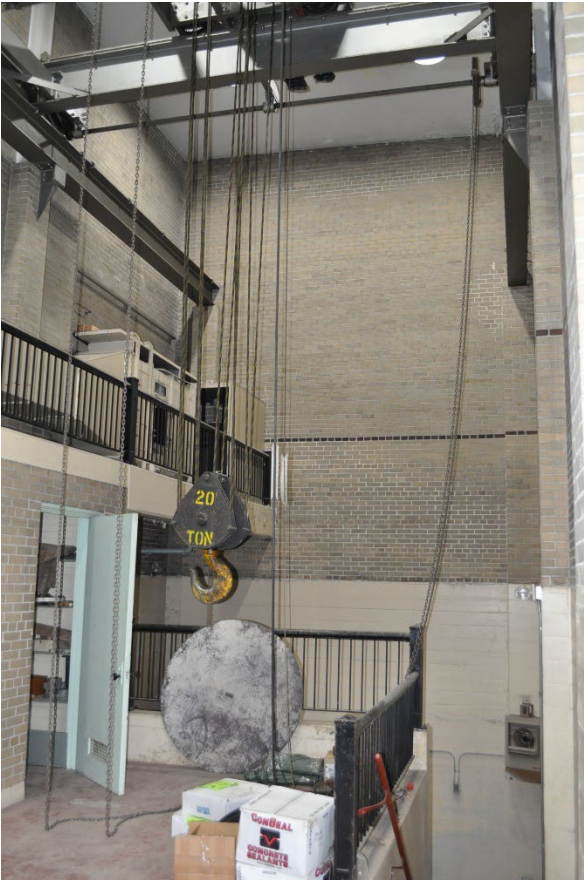
Storage Area and Crane
