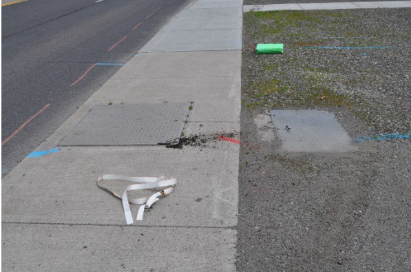
Grace Flowmeter Vaults
