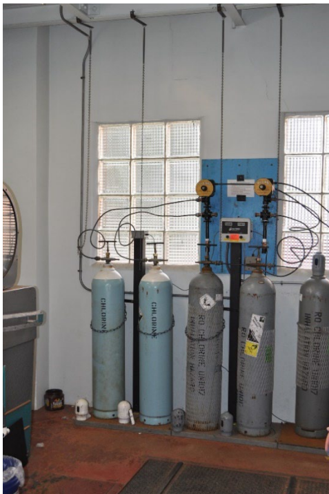
Gaseous Chlorine Tanks
