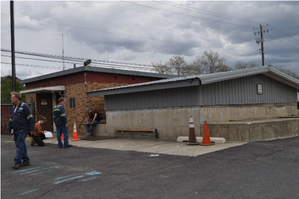
Nevada Pump Station and Chlorine Building Exterior
