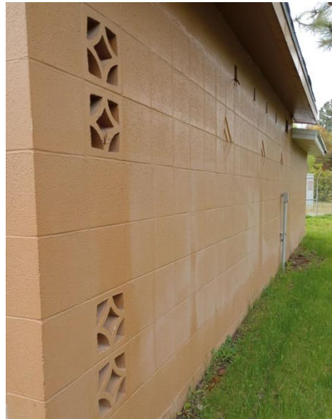
Figure 4-1 | Central Ave – CMU construction
