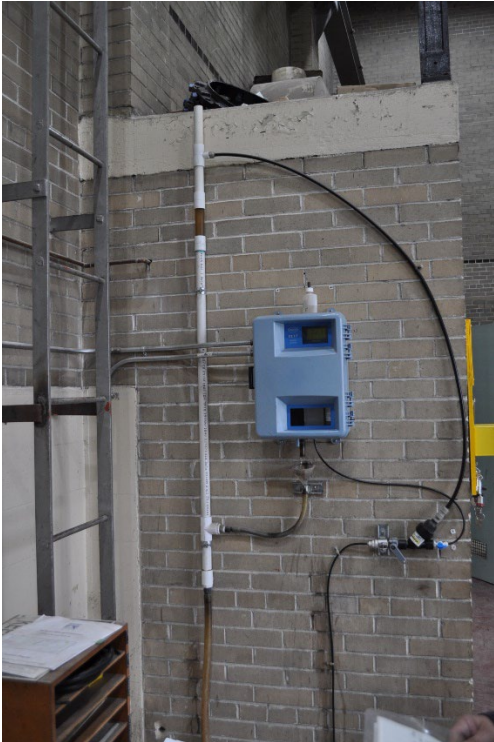
Hoffman Chlorine Analyzer
