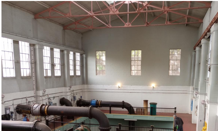
Figure 1-1 | Well Electric Well Station – Wells 4 and 5 Building Addition
