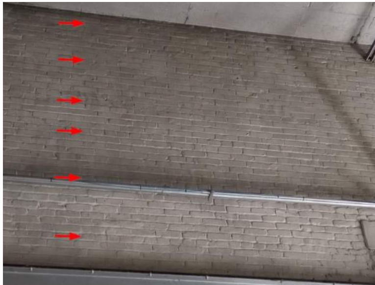
Figure 1-2 | Well Electric Well Station – Unreinforced Masonry ‘Header’ Course
