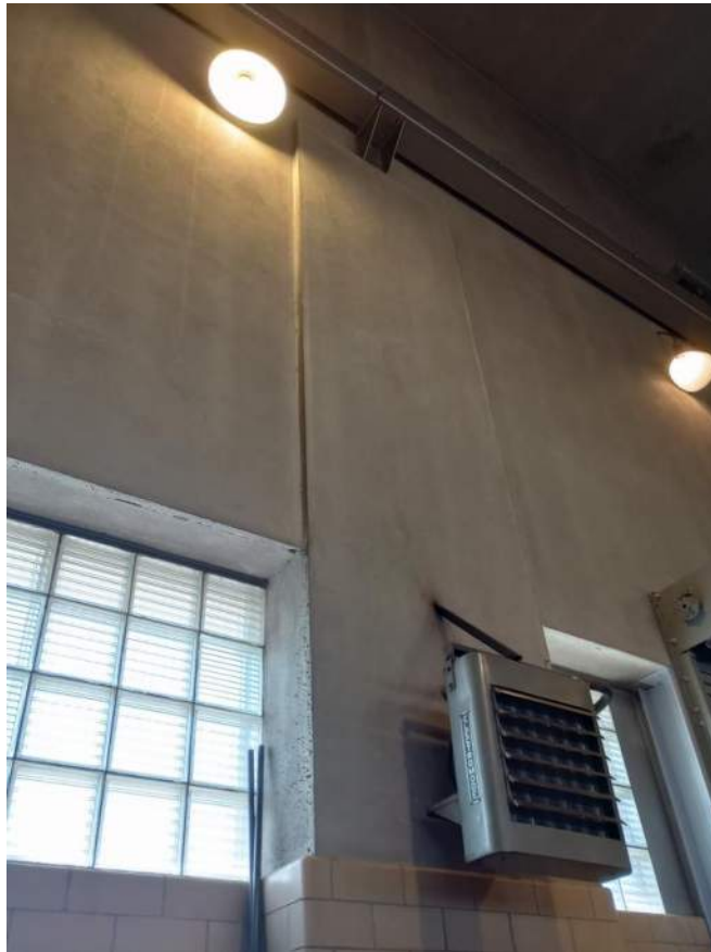
Figure 2-1 | Parkwater – Concrete Walls, Columns, and Ceiling
