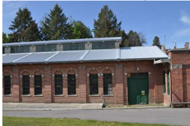
East Exterior of Well Building
