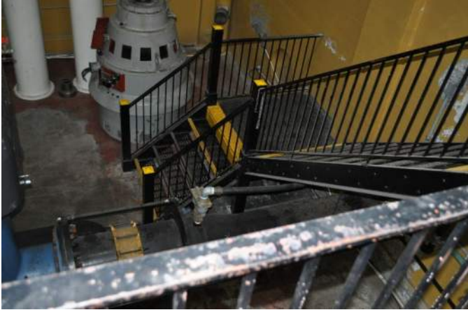
Future Pump Space
