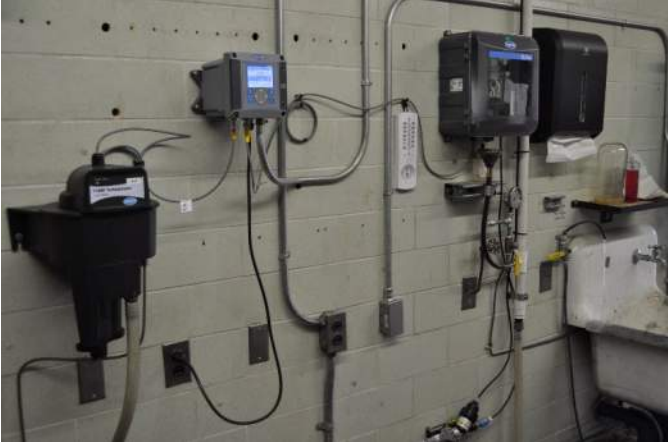
Nevada Turbidity and Chlorine Analyzer
