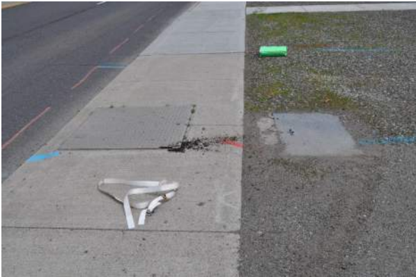
Grace Flowmeter Vaults
