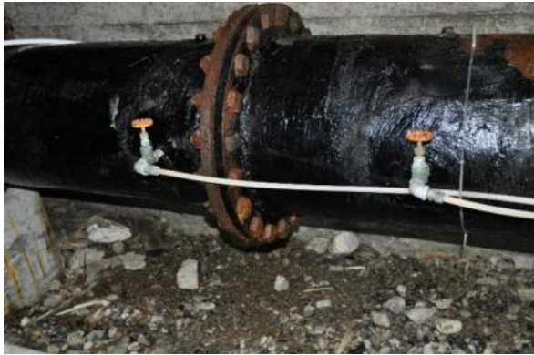
Differential Flow Meter
