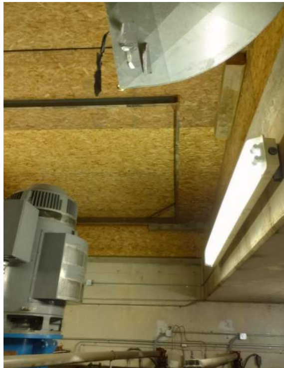
Figure 6-1 | Nevada – Concrete Walls and Timber Ceiling
