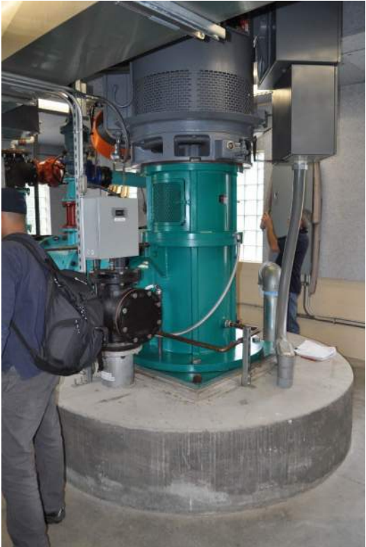
Well 1 Pump Motor
