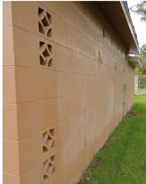
Figure 4-1 | Central Ave – CMU construction
