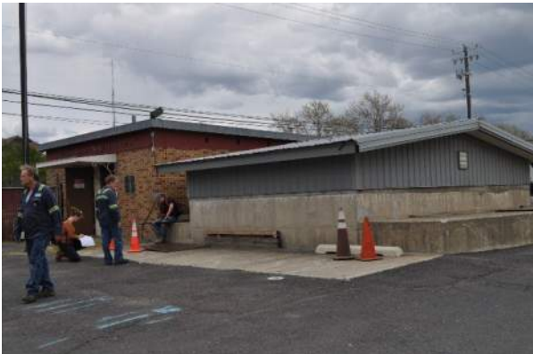
Nevada Pump Station and Chlorine Building Exterior
