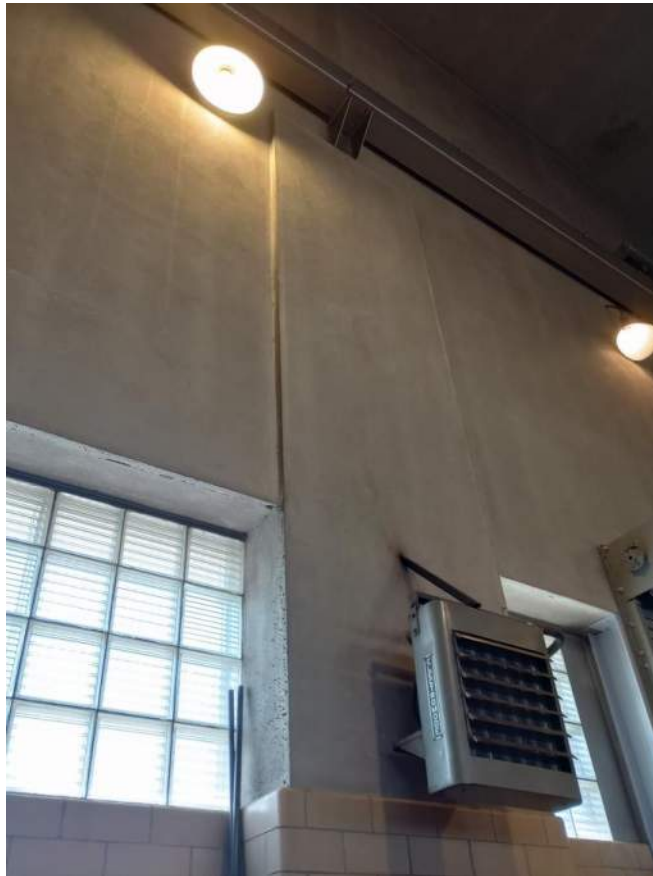
Figure 2-1 | Parkwater – Concrete Walls, Columns, and Ceiling
