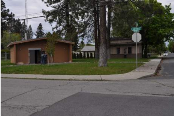
Control Building and Well 2 Building Exterior
