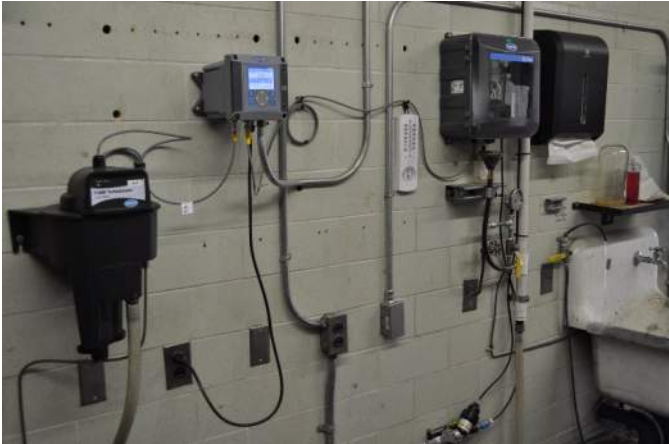
Nevada Turbidity and Chlorine Analyzer
