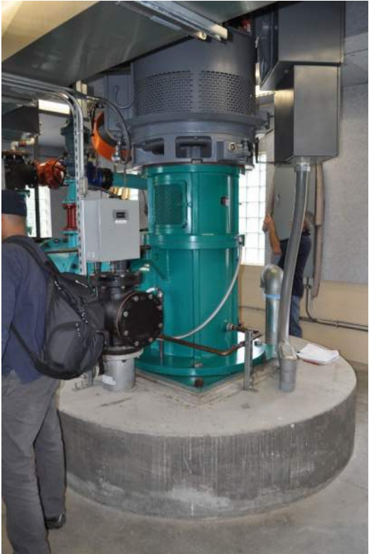
Well 1 Pump Motor
