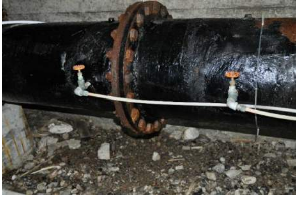
Differential Flow Meter
