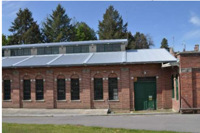
East Exterior of Well Building
