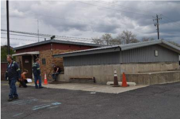
Nevada Pump Station and Chlorine Building Exterior
