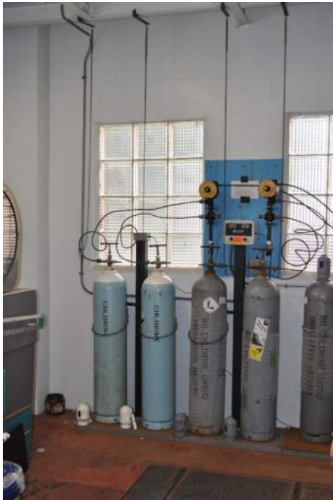
Gaseous Chlorine Tanks
