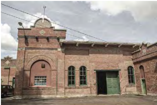
East Wing of Upriver Water Facility Looking North.jpg
