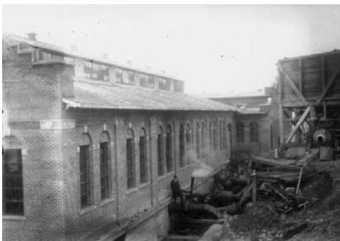
Well Electric Nearing Completion Looking NW.jpeg
