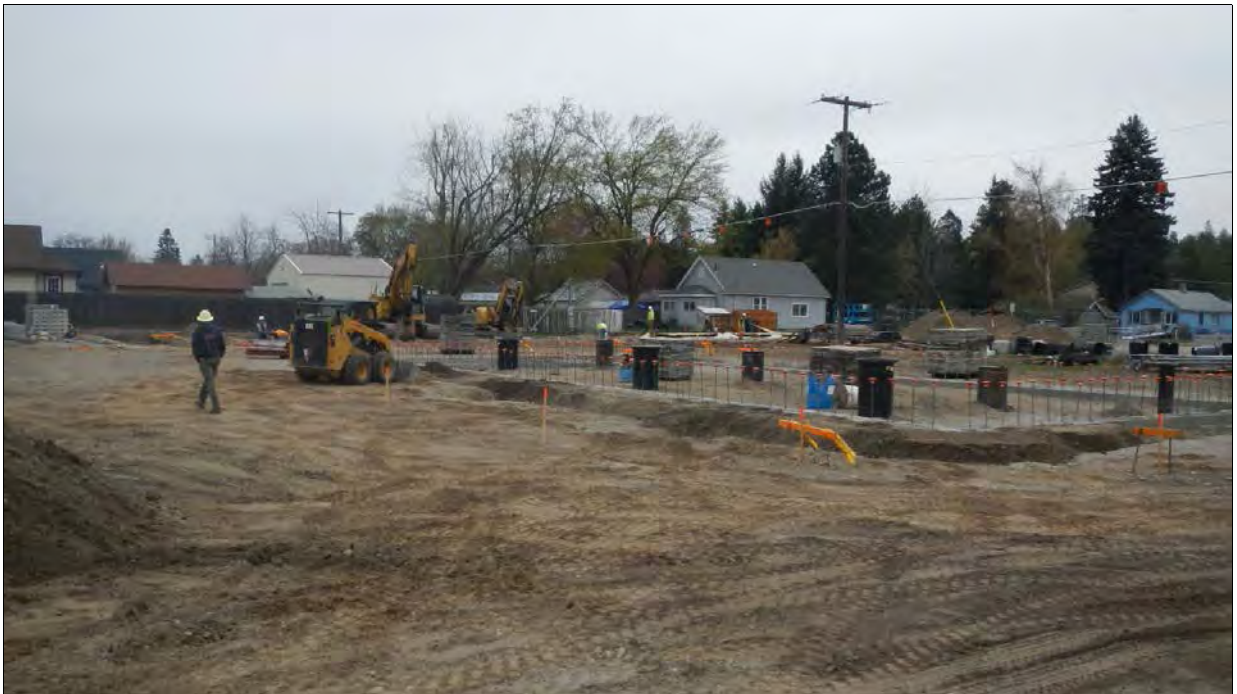
Figure 13. Havana Construction Site looking northeast.
