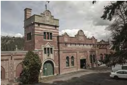
West Tower and Wing Upriver Water Facility Looking NE.jpg
