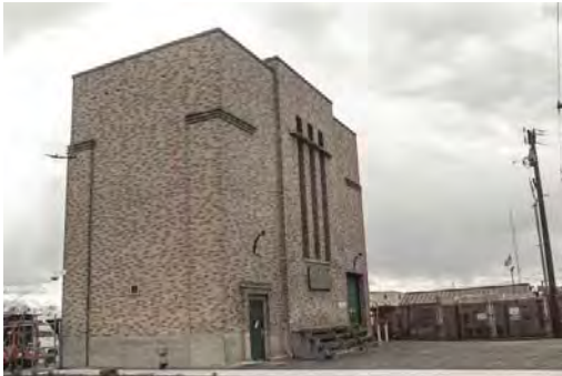
Grace Well Looking SW.jpg
