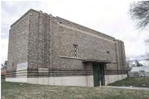
Hoffman Well Facade Looking NE.jpg
