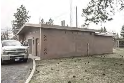
Central Well Looking South.jpg
