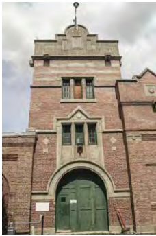
Central Tower Upriver Water Facility Looking North.jpg
