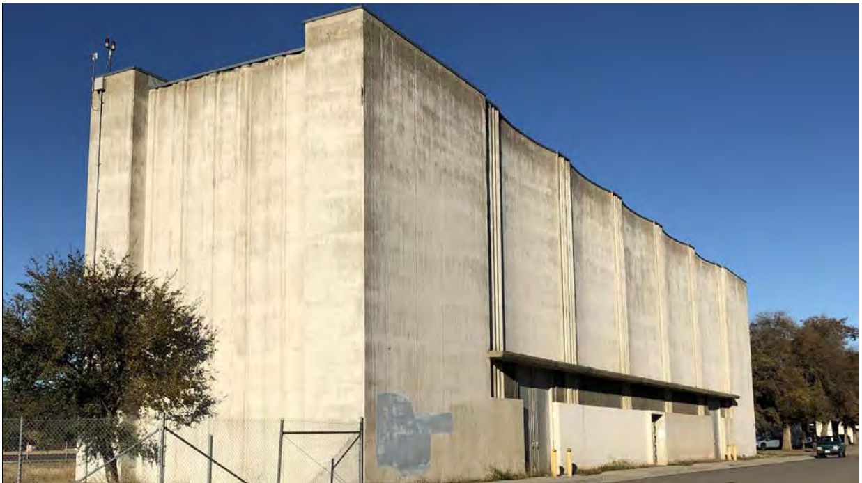
Figure 7. Parkwater pumping Station looking south.
