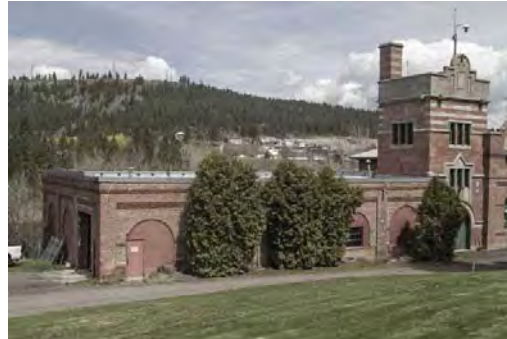
Far West Wing Upriver Water Facility Looking NE.jpg
