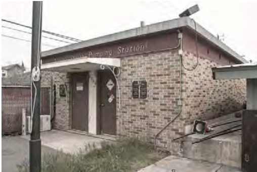
Nevada Well Control Structure Looking NE.jpg
