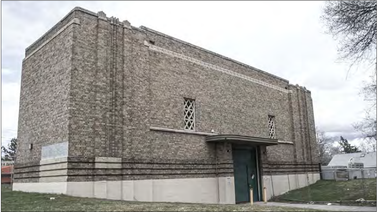
Figure 12. Hoffman Well Facade looking northeast.
