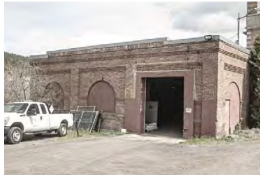
West Elevation Upriver Water Facility Looking NE.jpg
