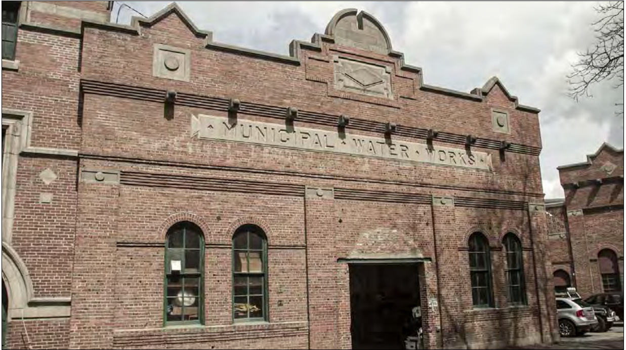
Figure 6. Upriver Water Facility looking north.
