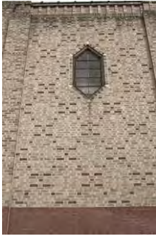
Ray Well with Garden Wall Pattern Looking East.jpg
