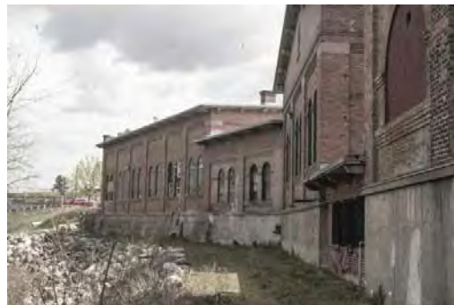
North Elevation Upriver Water Facility Looking East.jpg
