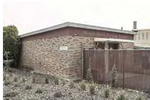
Nevada Street Well Control Room Looking SE.jpg
