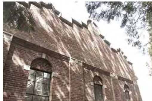
Well Electric SE Elevation Showing Raised Parapet.jpg
