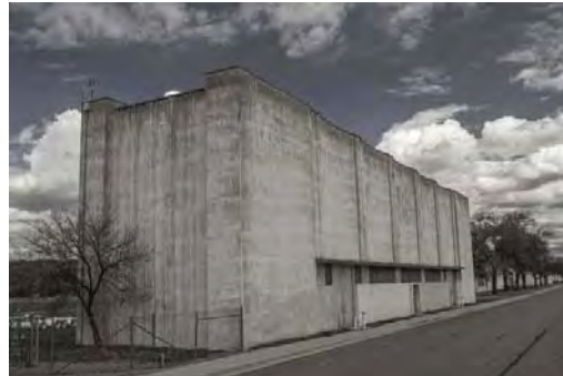
Parkwater Well South Elevation Looking NE.jpg
