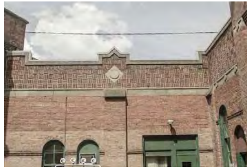
Triple Basket Weave Brick Detail Looking North.jpg
