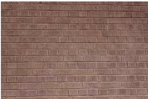
Ray Well Brick Bonding.jpg
