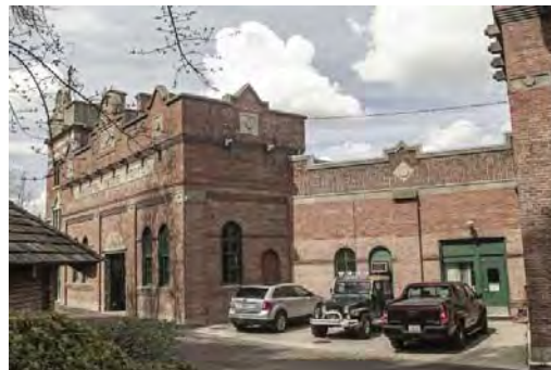
Central Wing Upriver Water Facility Looking NW.jpg
