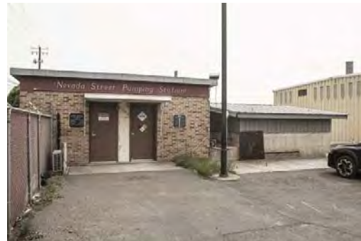
Nevada Street Control Room and Well Structure Looking East.jpg
