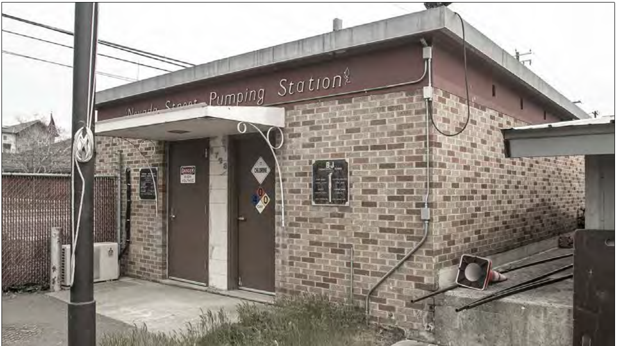
Figure 11. Nevada Well Control looking northeast.
