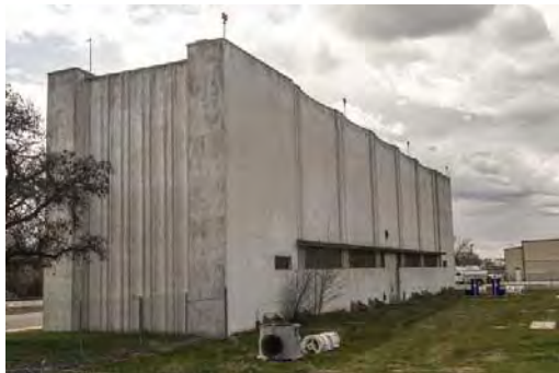
Parkwater Well East and North Elevation Looking SW.jpg
