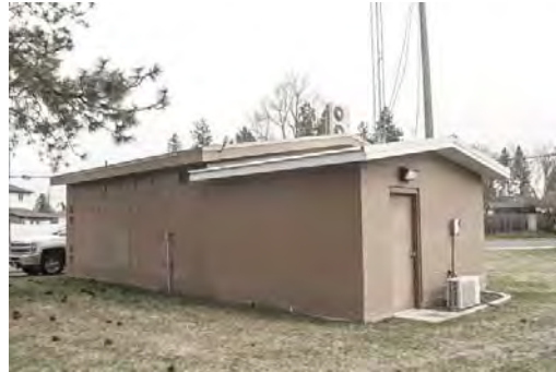
Central Well with 2014 Addition Looking SE.jpg
