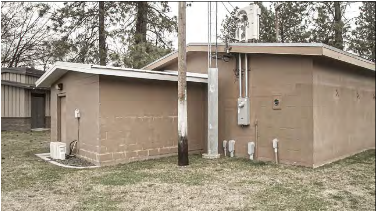
Figure 9. Central Well with 2014 addition looking northeast.
