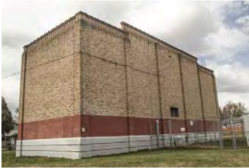
Ray Well South and East Elevations Looking NW.jpg
