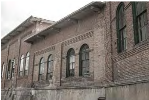
North Elevation Upriver Water facility Looking SE.jpg
