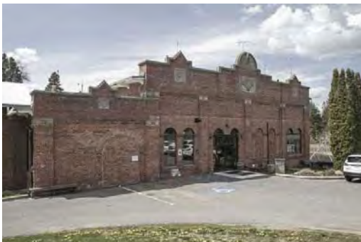
East Elevation Looking NW.jpg
