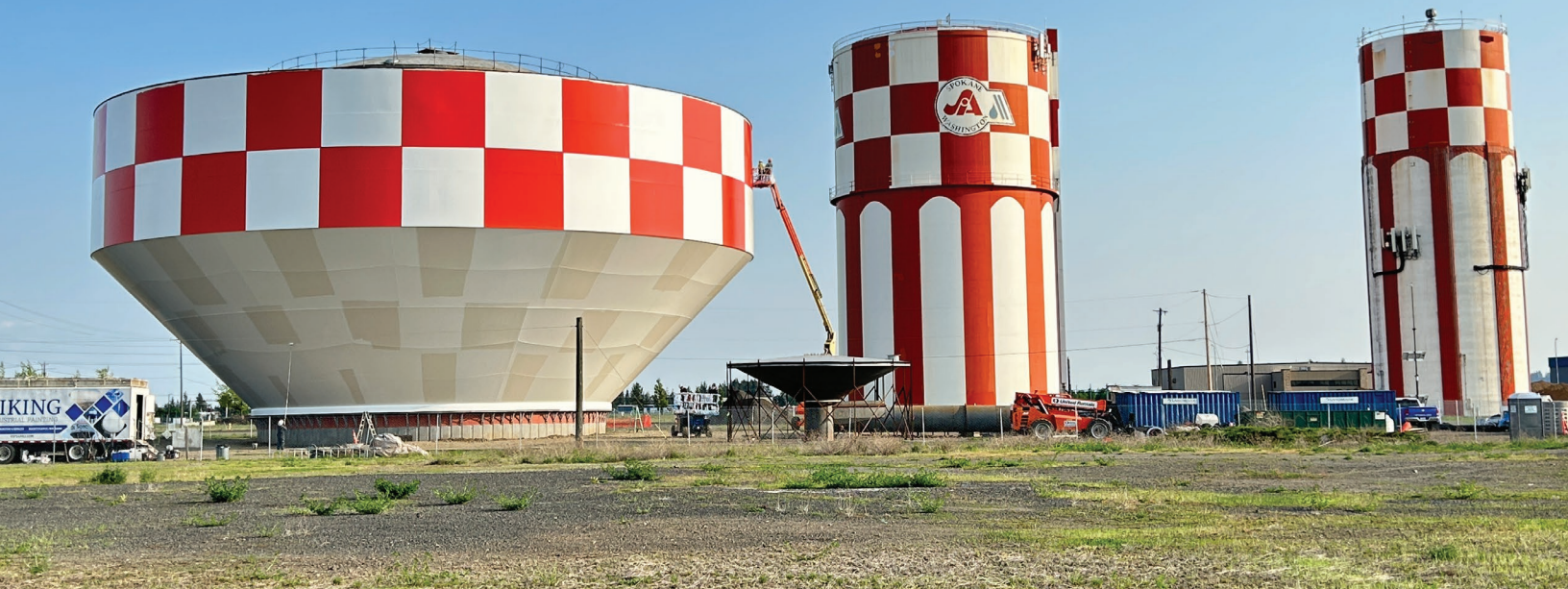
The additional reservoir under construction at the Spokane International Airport will add 4.2 million gallons of water storage to the system.
