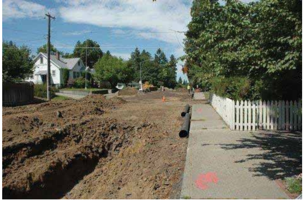
Integrated utility improvement project on 29th Avenue, in 2012
