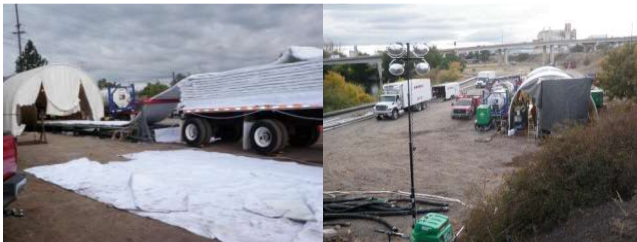
FIGURE 2-4: CURED IN PLACE PROJECT FOR STRUCTURAL REHABILITATION OF 60" LINE TO PREPARE FOR NEW MLK JR. WAY
