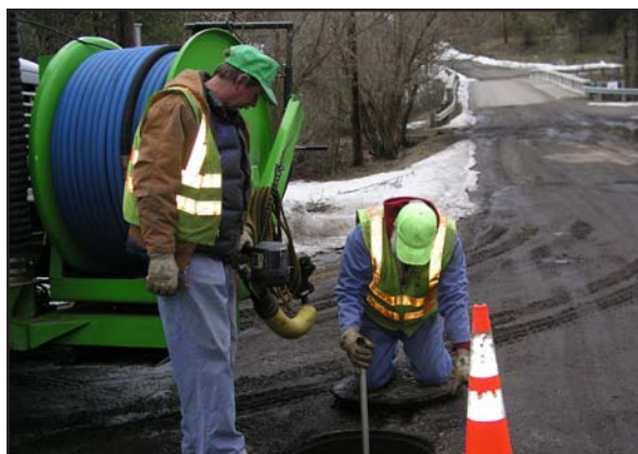
Vactoring pipelines free of debris
