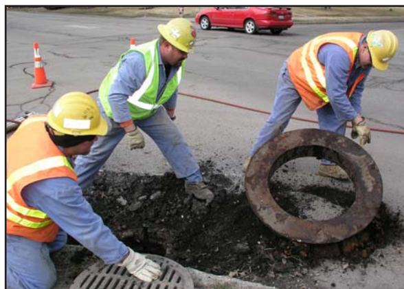
Replacing a manhole cover
