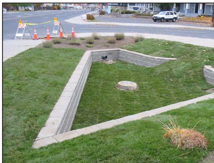
Bio-Infiltration Swale at Northwest and Knox Street
