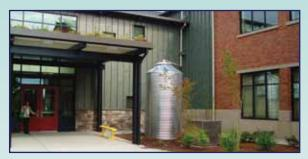
Capturing roof runoff in a cistern or rain barrel allows for reuse for irrigation.
