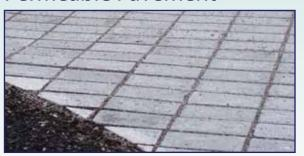
Pavement that allows water to move through it. Some options include interlocking concrete pavers, pervious concrete, and porous asphalt. Permeable pavement is applicable to low-traffic areas such as parking areas and sidewalks.
