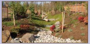
Open conveyance may reduce the size of or entirely eliminate conventional underground piped conveyance systems.
