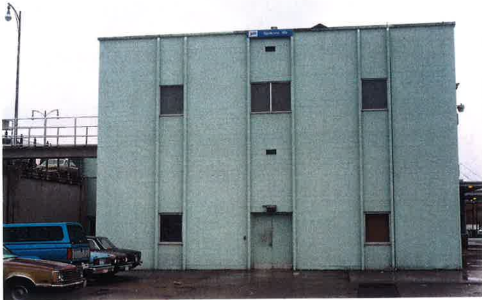
3. EAST SIDE OF DEPOT BUILDING
