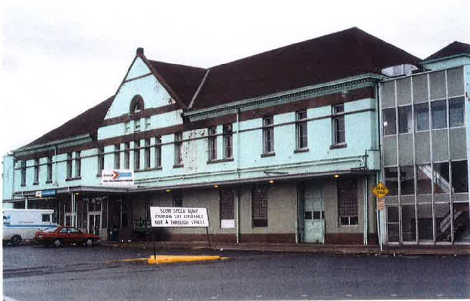
1. NORTH SIDE OF DEPOT BUILDING
