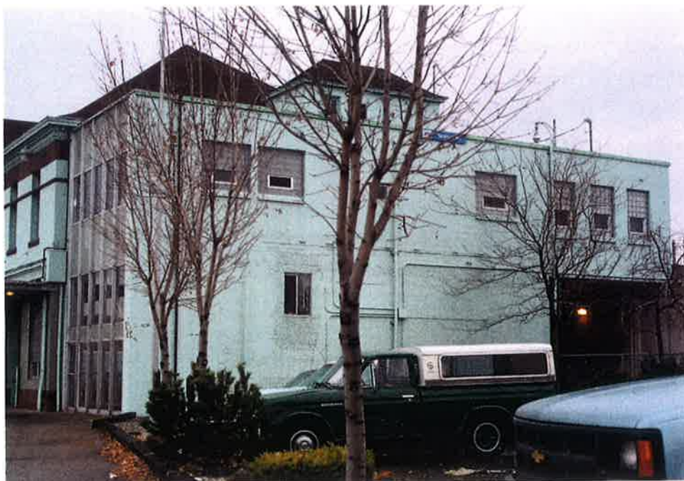
2. WEST SIDE OF DEPOT BUILDING
