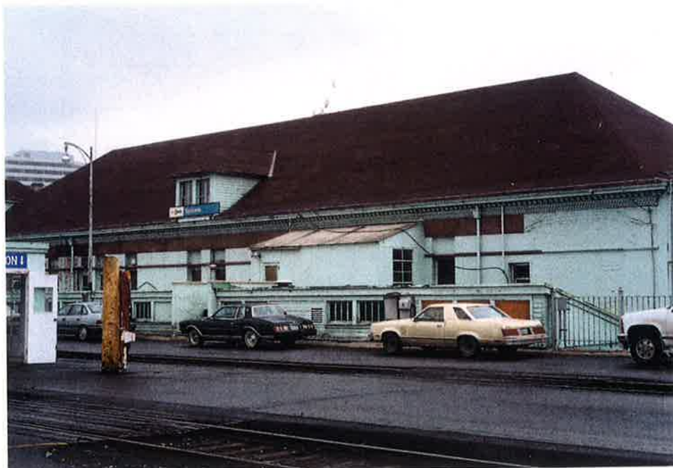
4. SOUTH SIDE OF DEPOT BUILDING
