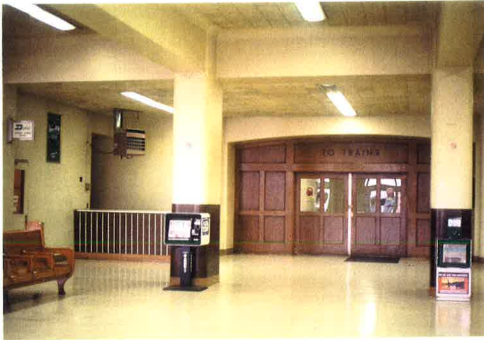
7. PASSENGER WAITING AREA AND BOARDING ENTRANCE - FIRST FLOOR OF DEPOT BUILDING LOOKING SOUTH
