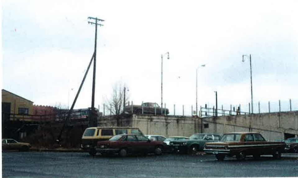
12. ADJACENT PROPERTY EAST OF DEPOT BUILDING
