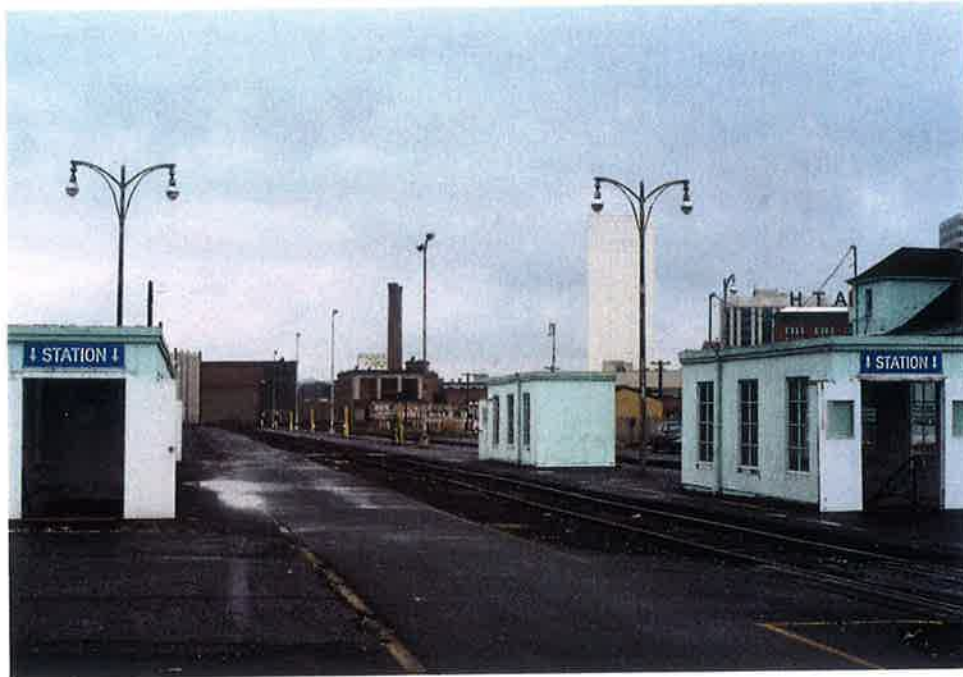
5. RAILROAD TRACKS AND PASSENGER ACCESS TO STATION - SOUTH SIDE OF DEPOT BUILDING LOOKING WEST
