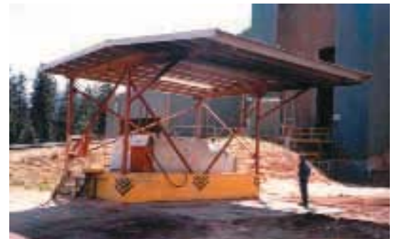
Figure 12 On/off loading pad with blind sumps.
