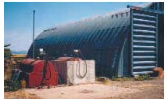
Figure 13 Small on/off loading pad with blind sump.
