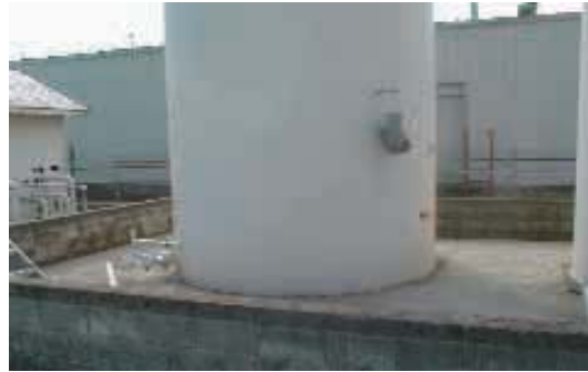
Figure 1 Concrete Block Secondary Containment
