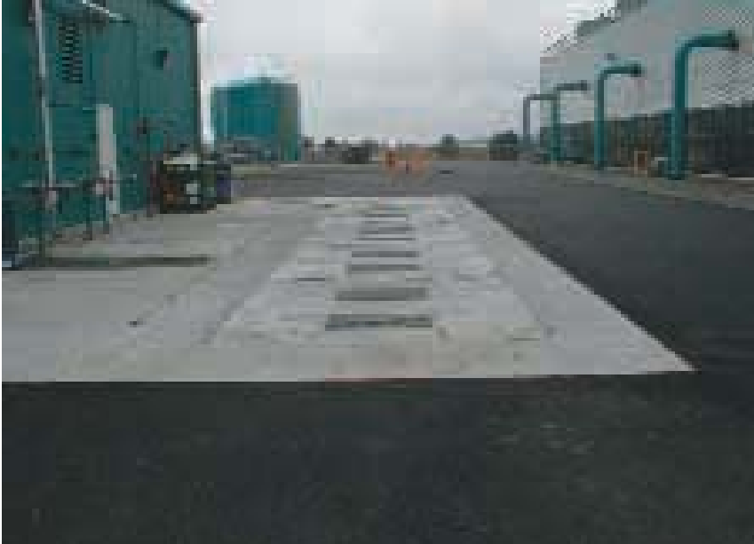
Figure 7 Loading platform that slopes to the center.
