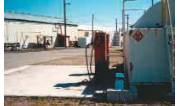
Figure 11 trench located in shaded area of pad.
