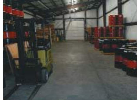
Figure 3 Concrete Floor Sloped to Center
