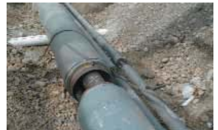
Figure 19 Example of double wall piping.
