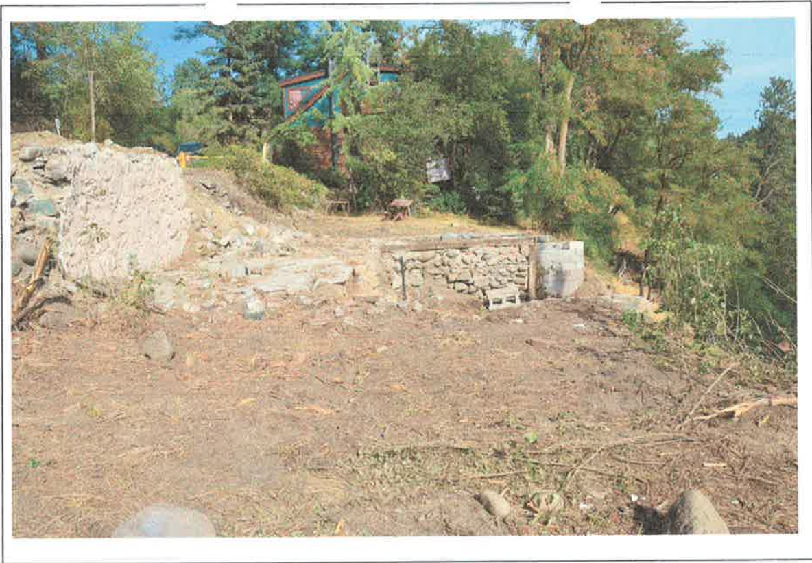
Photo 3 – View to East Across Flat Bench Showing Foundations of Former House (Steep Slope to South Toward River Shoreline)
