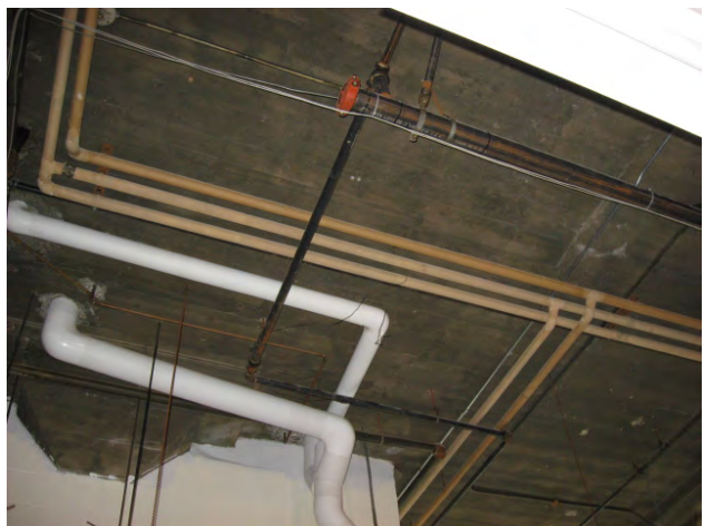
TYPICAL INTERIOR PIPING INSULATIONS PRESENT WITHIN THE 3-STORY BUILDING AREA OF THE FACILITY
