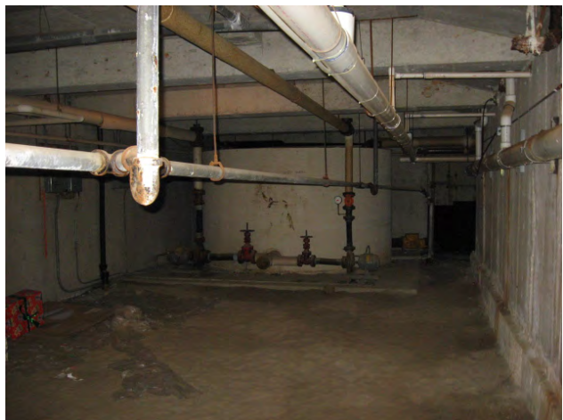
TYPICAL VIEW OF THE SWIMMING POOLS BASEMENT MECHANICAL CRAWL SPACE & WELL WATER HOLDING TANK ALSO JACKETED WITH ASBESTOS INSULATION
