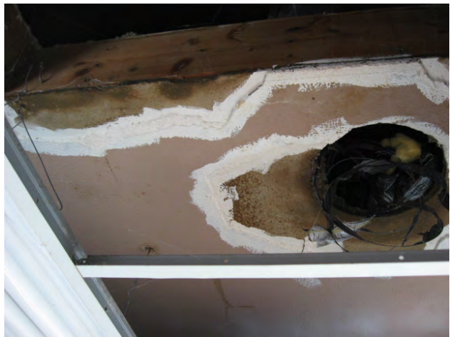
VIEW OF THE HIDDEN ACM BROWNS-COAT CEILING TEXTURE PRESENT WITH THE 2 ND FLOOR OFFICES AREA OF THE CENTRAL CORE BUILDING AREA OF THE FACILITY
