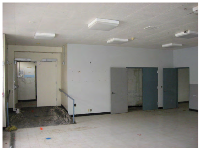
VIEW OF THE CENTRAL CORES, ENTRY LOBBY ROOM & ACCESS TO THE 3-STORY BUILDING AREA OF THE FACILITY; CEILING TILE, FLOOR TILE & HIDDEN STEAM PIPING SYSTEMS ARE REGULATED ACMs
