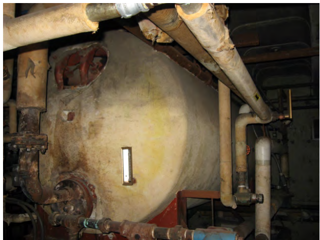
INTERIOR VIEW OF A TYPICAL WATER HOLDING TANK THAT COVERED WITH AN ASBESTOS JACKET TYPE INSULATION
