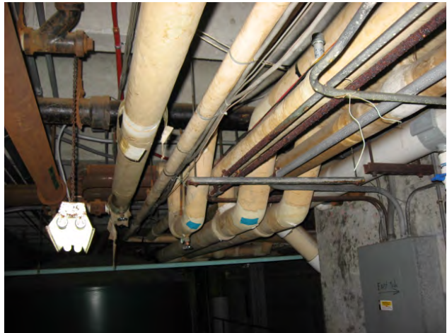
VIEW OF THE TYPICAL INTERIOR STEAM & DOMESTIC WATER PIPING INSULATIONS PRESENT THROUGHOUT
