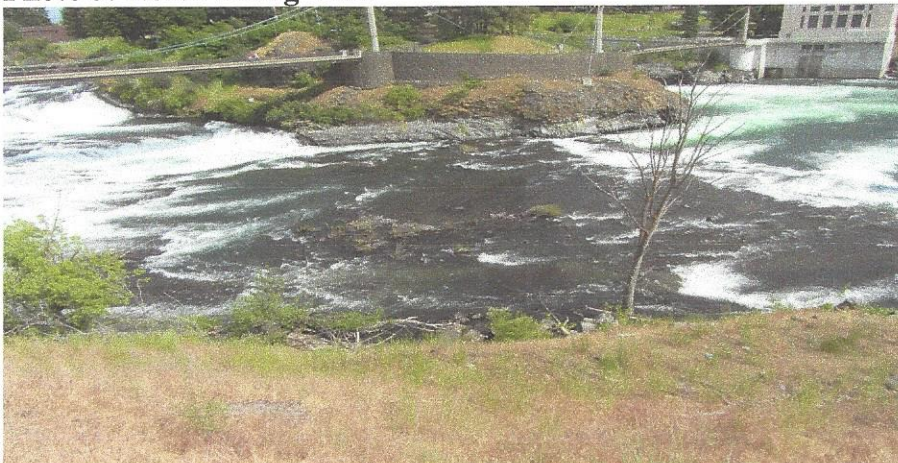
Photo 4: East Facing View
