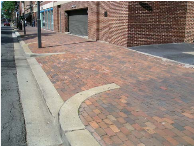
Figure 13 - Brick sidewalk pattern is continued over the driveway to establish pedestrian dominance.
