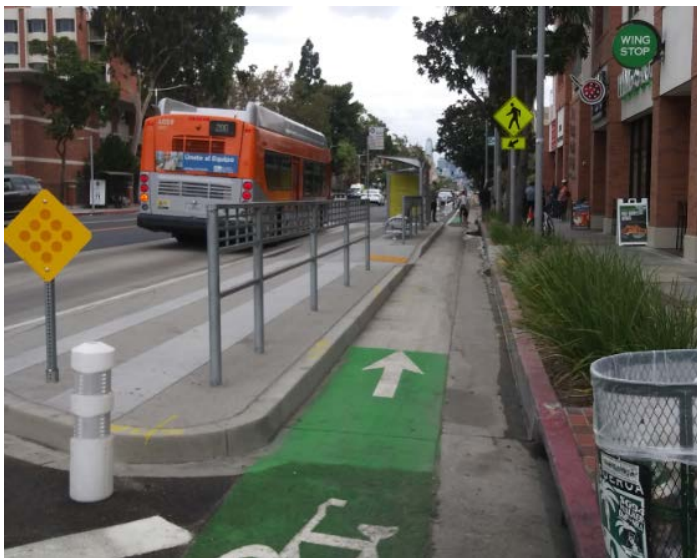
Figure 9 – Island bus stop separates bike lane from bus traffic
