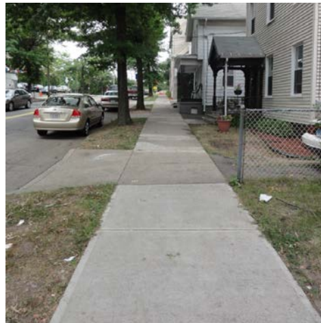
Figure 18 - Continuous Sidewalk Design Establishes Pedestrian Space over Driveway
