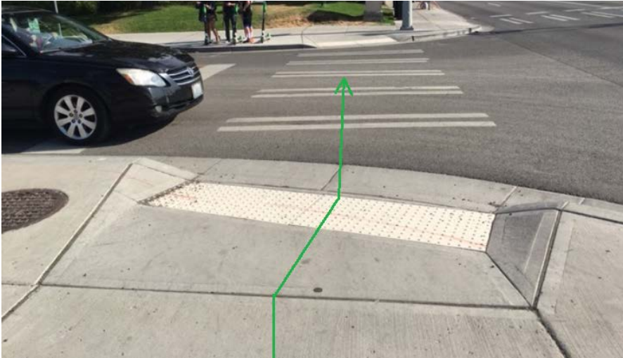
Figure 7 – Ramp running slope misaligned with crosswalk does not provide information to sight impaired individuals
