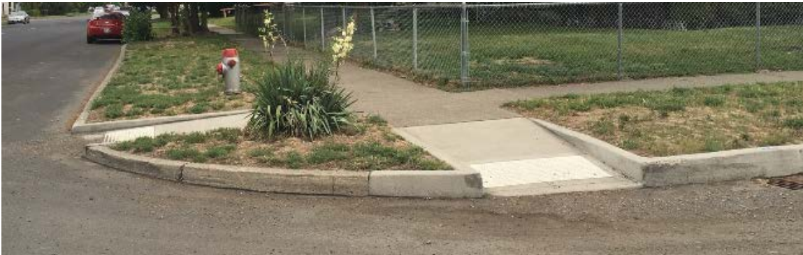
Figure 8 – Dual ramps with curbs instead of flares
