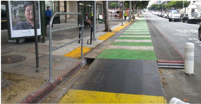
Figure 10 – Shared bike lane and bus stop using temporary platform
