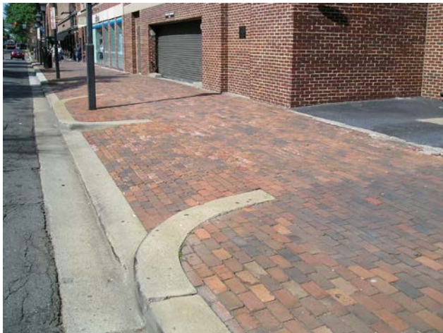
Figure 17 - Brick sidewalk pattern is continued over the driveway to establish pedestrian dominance.
