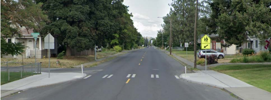
Figure 5 – Curb extension works to narrow a road adjacent to a school
