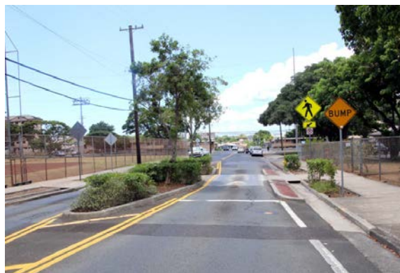
Figure 9 – Midblock curb extension works to narrow a road adjacent to a school without moving existing curbs
