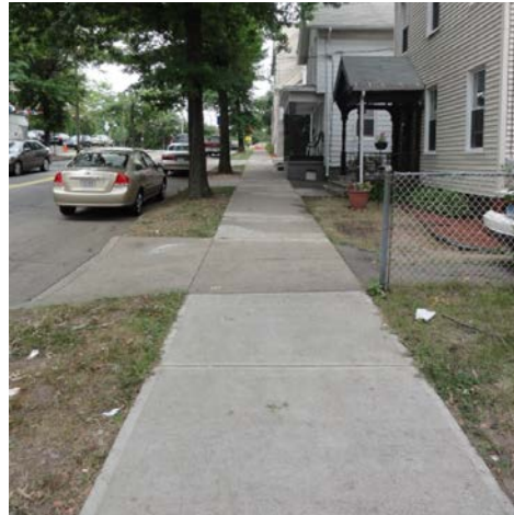
Figure 16 - Continuous Sidewalk Design Establishes Pedestrian Space over Driveway
