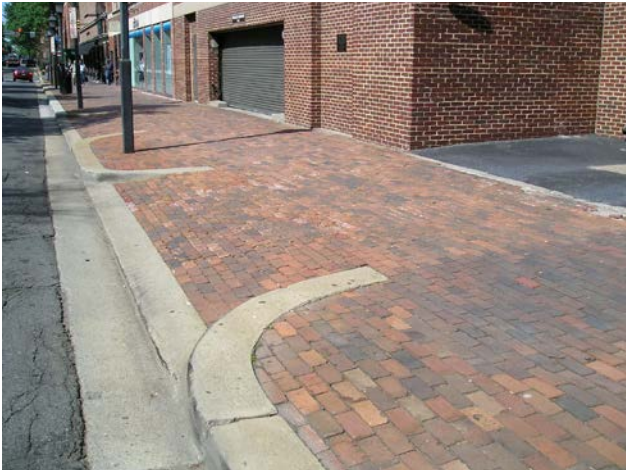
Figure 15 - Brick sidewalk pattern is continued over the driveway to establish pedestrian dominance.
