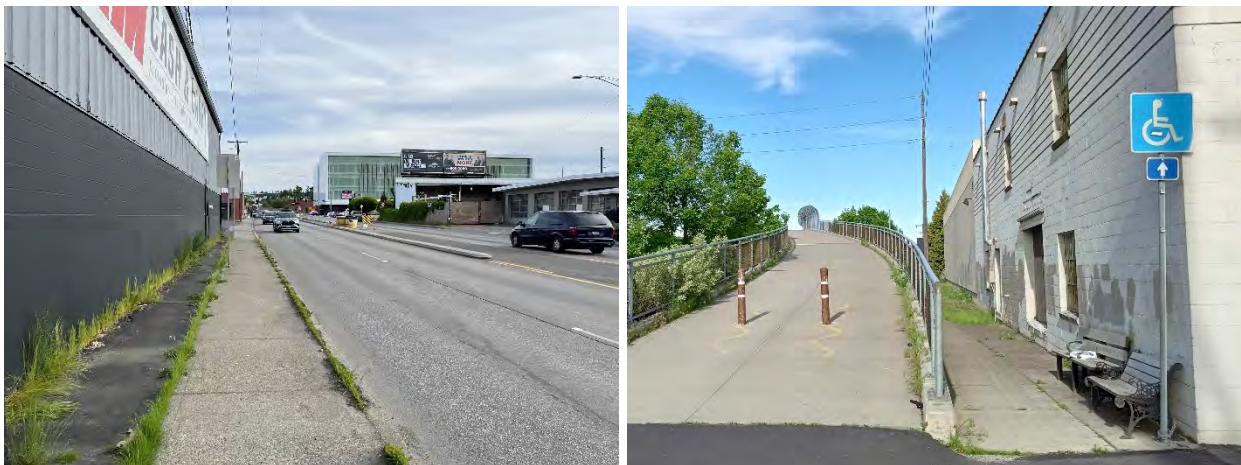
Figure 15. Left: A narrow sidewalk next to high-speed traffic on Hamilton St creates an unnerving walking environment. Right: The Centennial Trail bridge over Hamilton St is too steep to provide an ADA compliant pathway.
