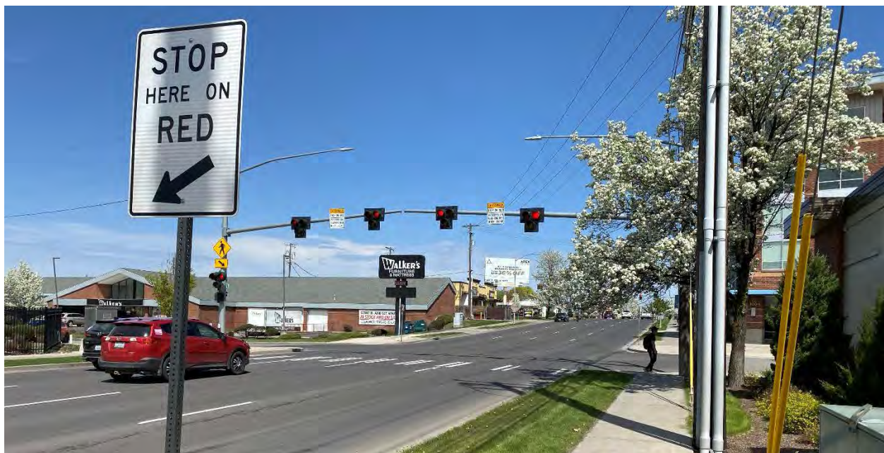
Figure 42. Crosswalk with a HAWK signal on Ruby Ave in Spokane.
