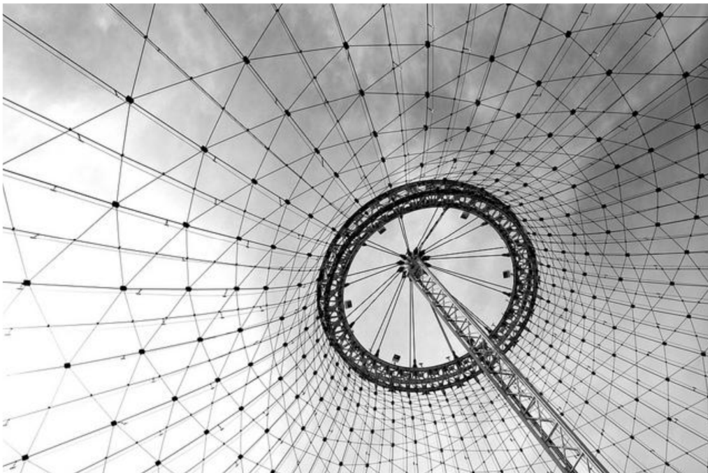
Photo 6: Cable structure of United States Pavilion (Photo came from Riverfront Park Master Plan, 2014)
