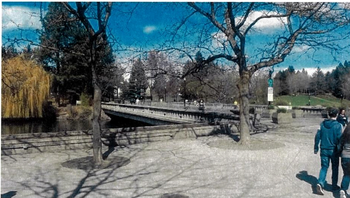
Photo 2: At southwest corner of the Howard Street South Channel Bridge looking towards the northwest corner, which is the only bridge riverbank with native soil/vegetation to river's edge. Riverbanks at remaining corners of the bridge have concrete walls and concrete/asphalt ground surfaces.
