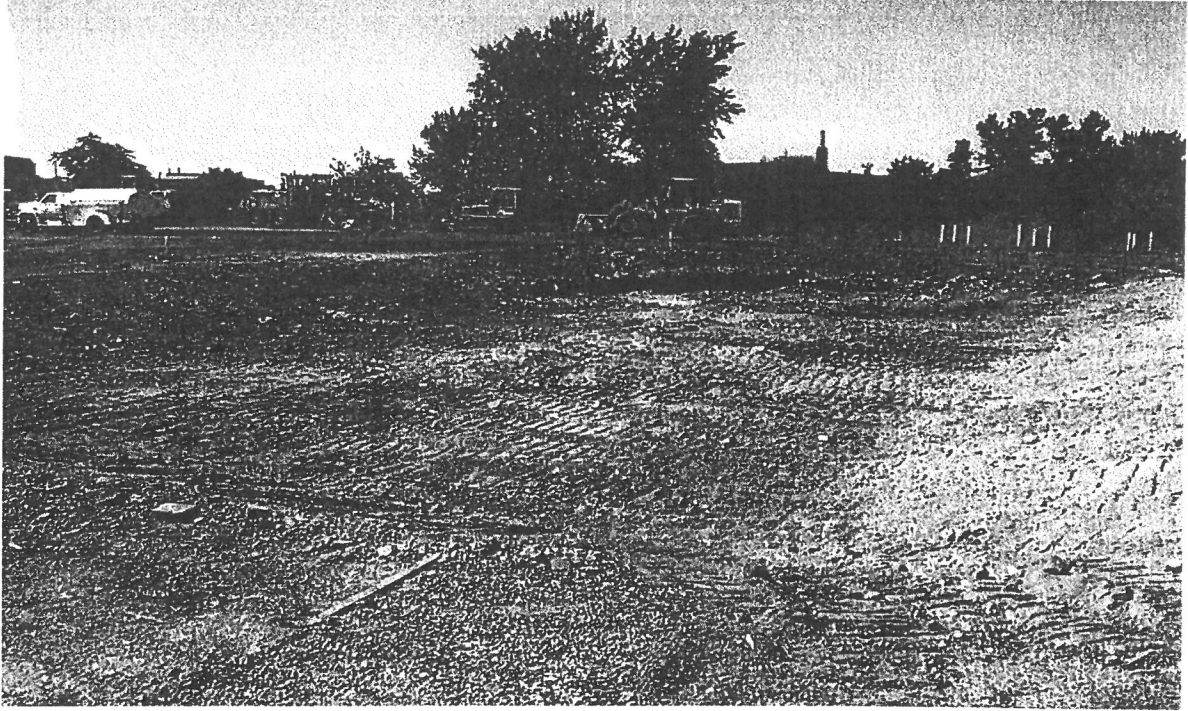
View of west detention basin (looking northwest).
