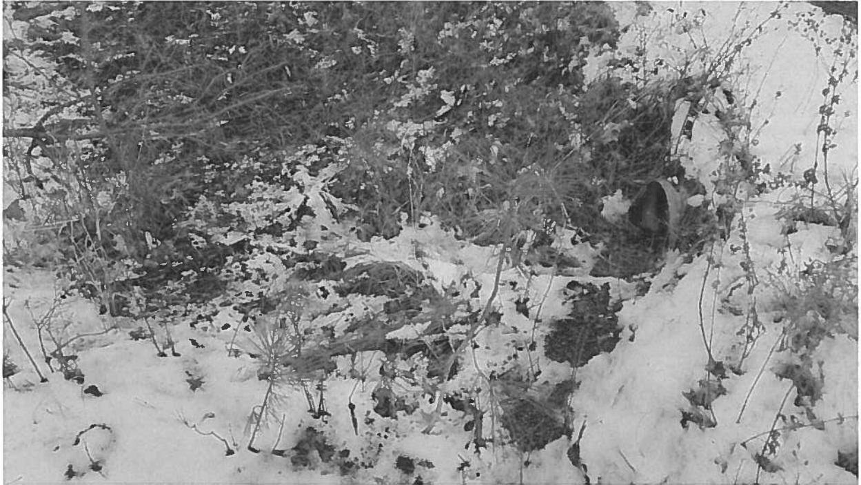
Photo 5: Stream B culvert under private driveway, upstream end.
