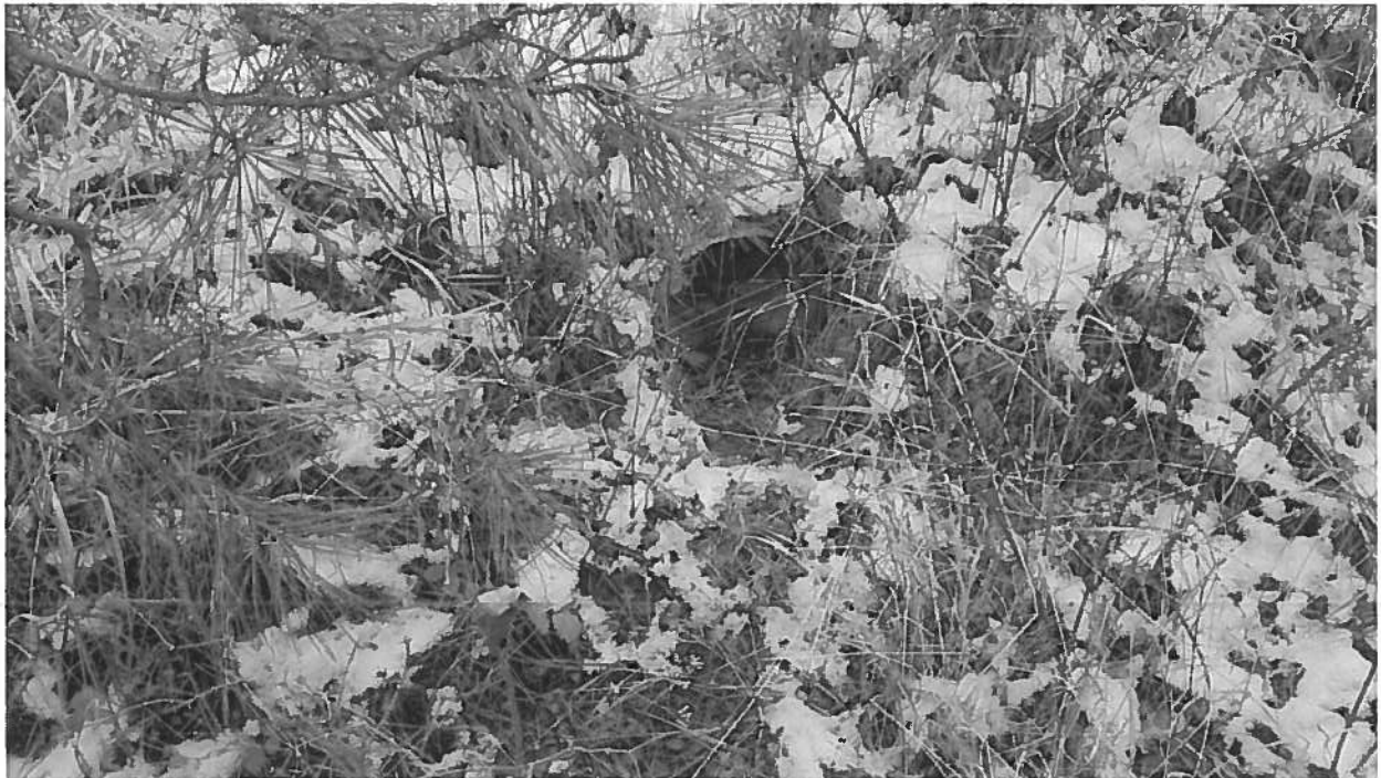
Photo 6: Stream B culvert under private driveway, downstream end.
