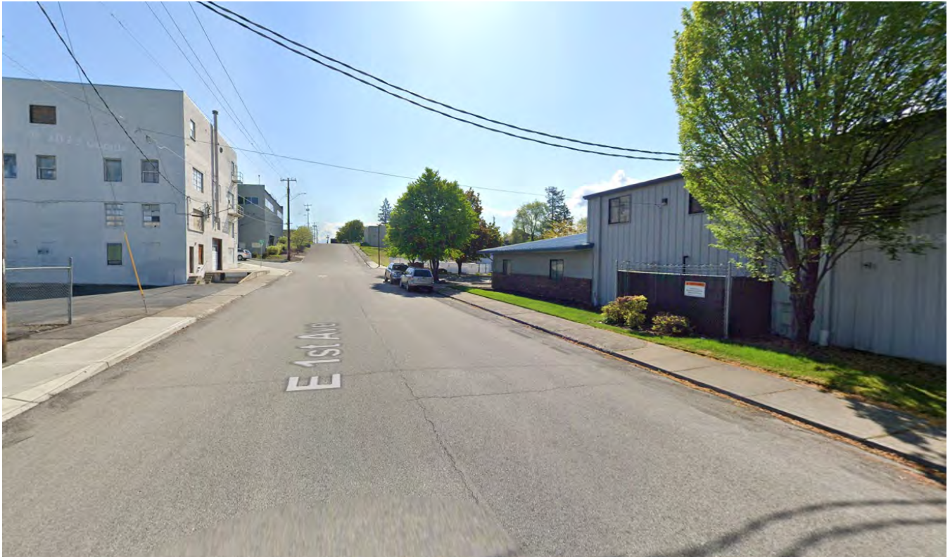
Figure 23: E 1 st Ave, looking East towards S Ivory St (From Google Street View)
