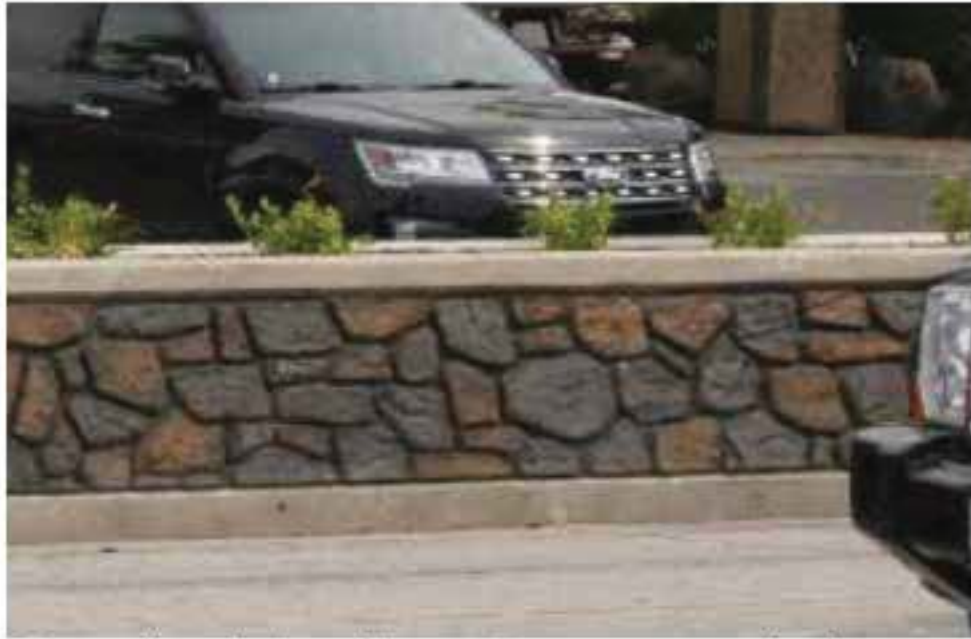
Standard Aesthetic Barrier and planter on Division. Texture and surface stain.
