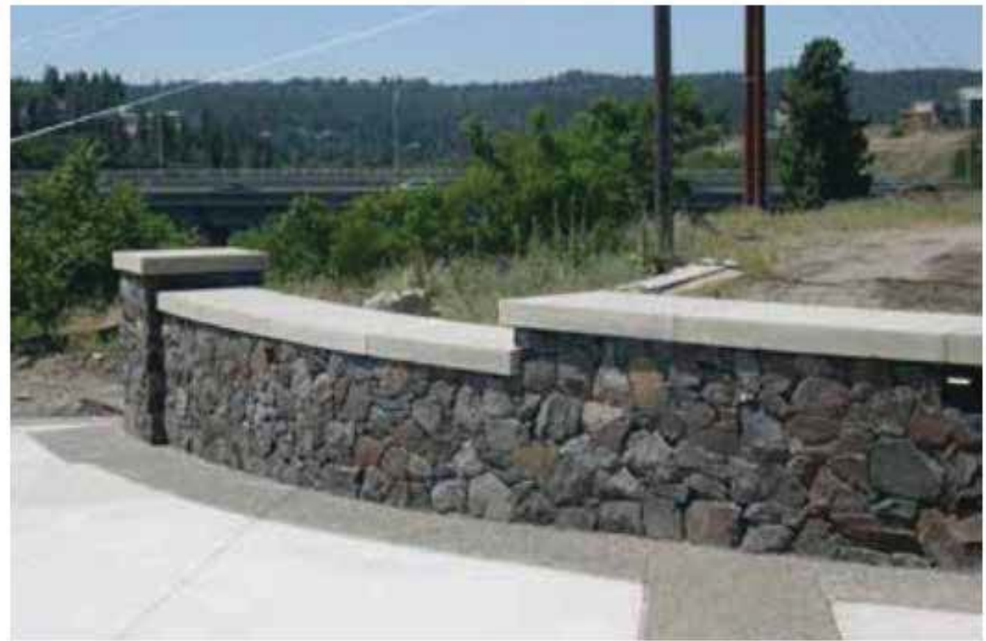
Recently installed basalt wall at Kendall Yards.
