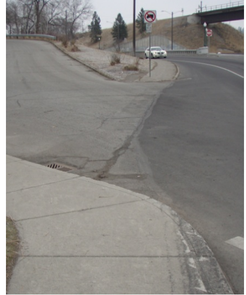
Curb ramps are missing from the intersection of Coeur d'Alene Street and Sunset Boulevard.
