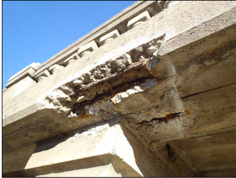
Photo C2-03 (ID C101) – Deterioration between Floorbeams 18 and 19 along south overhang in Span 3.
