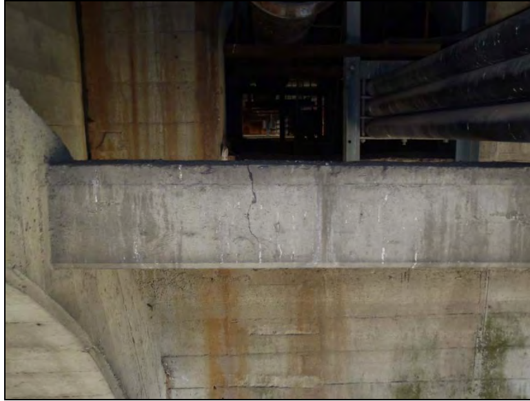
Photo C3-109 (ID C271) – Transverse beam between Spandrel Arches C & D at Floorbeam 27. Vertical crack 2' from face of Spandrel Arch C. This cracked condition is typical at several locations
