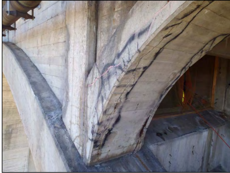
Photo C3-70 (ID C247) – Span 3, Spandrel Arch D, between Floorbeams 20 & 22. Large delaminated areas with exposed bars and rust staining on both corners. Typical at symmetrical locations.
