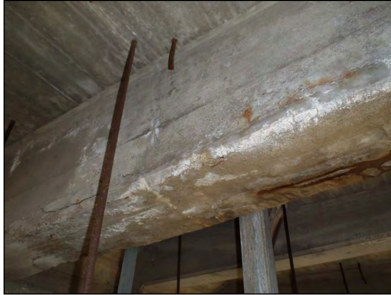
Photo C3-90 (ID C257) - Span 3, Floorbeam 24 between arch rib lines C & D. Entire bottom face is delaminated. Extensive evidence of rust staining and seepage through joint.
