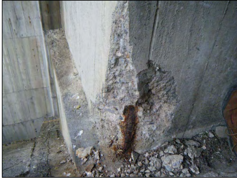
Photo D1-06 (ID D007) – Span 3, Spandrel Column B-24, large corner spall with exposed reinforcing steel with 1/16” loss to bar.
