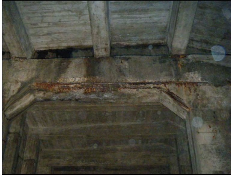
Photo D2-07 (ID M101) – Large spalled area with exposed bottom bars on floorbeam where East Approach meets Arch Span 1. Water leakage through joint above.
