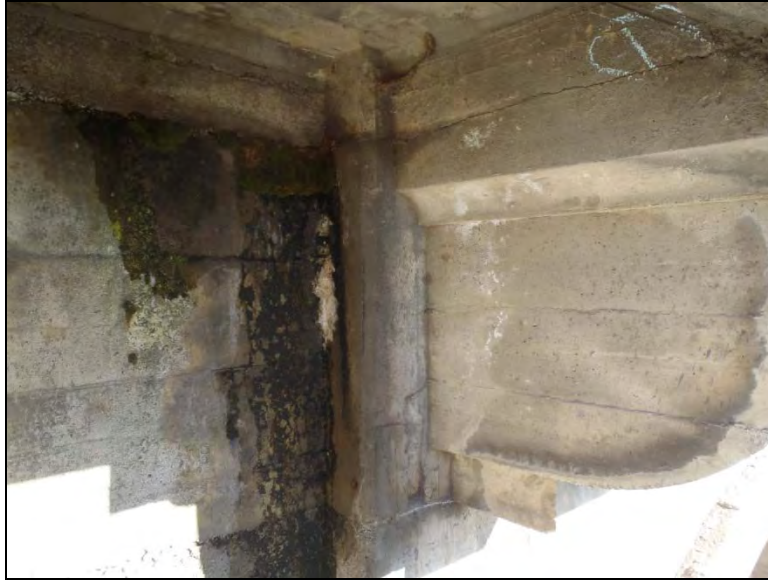
Photo C2-22 (ID C121) – South sidewalk overhang at Floorbeam 8. Evidence of leakage through joint and 6" dia. delaminated area.
