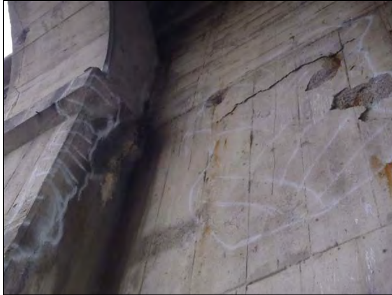
Photo C1-13 (ID C008) – West face of Pier 3 between Arch Ribs A & B. 4' x 6' delaminated area and 6' high corner delamination on pilaster above Arch Rib A. Localized spalls are present in the delaminated areas and have exposed bars with up to 1/8" loss to bar diameter.
