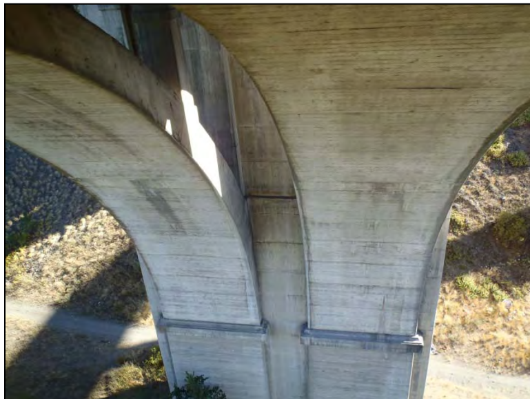
Photo C2-25 – Typical condition of arch soffit in Span 3
