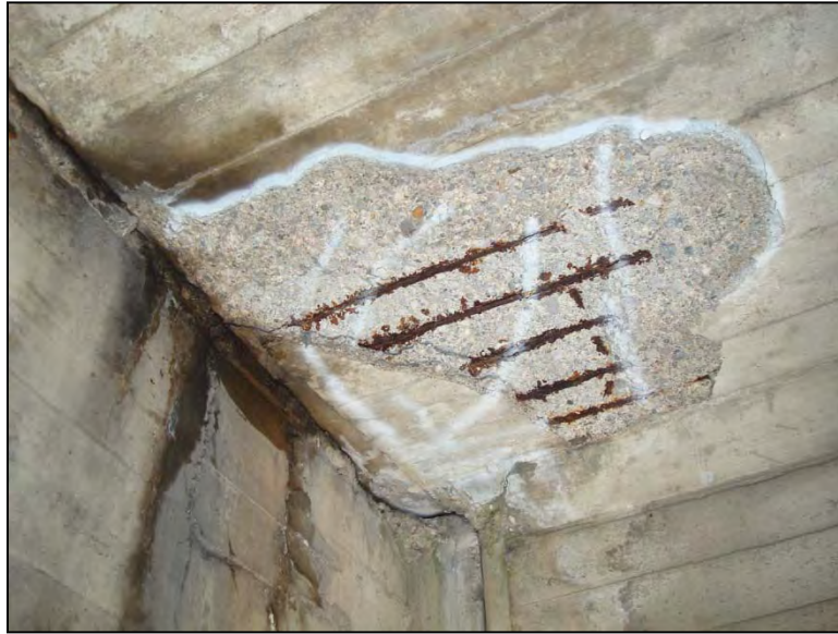
Photo C4-38 (ID C325) – Soffit between west face of Pier 2 and Floorbeam 1 in Span 3, 5' x 5' area of spalling, delamination and exposed rebar, 3/8" diameter remaining on rebar.
