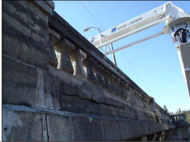
Photo C3-61 (ID C244) - North exterior rail between Floorbeams 16 & 18, Span 3, wide horizontal cracks in rail both above and below balusters.
