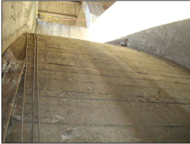
Photo E2-10 –Typical overall view, arch floor between Arch Ribs A & B below Floorbeams 1-4. Note typical rough/poor formwork/finishing and localized honeycombing patches.
