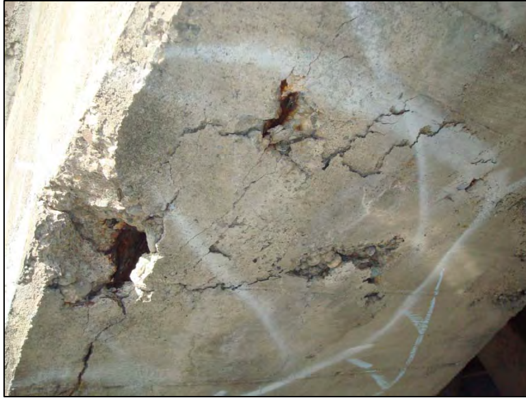
Photo C4-17 (ID C311) – Span 3, Spandrel Arch A soffit, between Floorbeams 2 & 3. 5' H x 4' W x 4" D delaminated area with spalls and exposed reinforcing steel. Bars exhibit approximately 3/16" section loss maximum.
