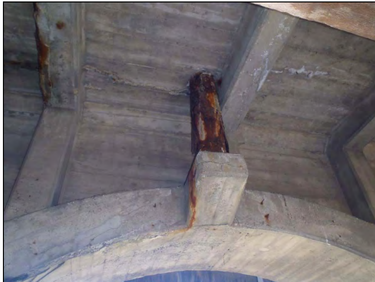
Photo C3-31 (ID C223) – Light pole pilaster at Floorbeam 6. Corrosion related distress to steel pole and concrete pilaster.
