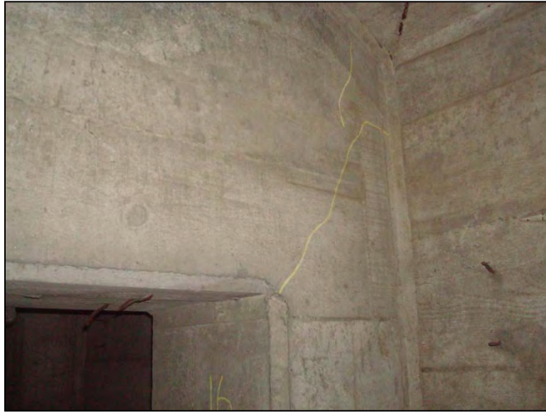
Photo E1-03 (ID E004) – Narrow diagonal cracks at pilaster-floorbeam intersection. Typical both web faces. No exposed bars, leakage or rust staining.
