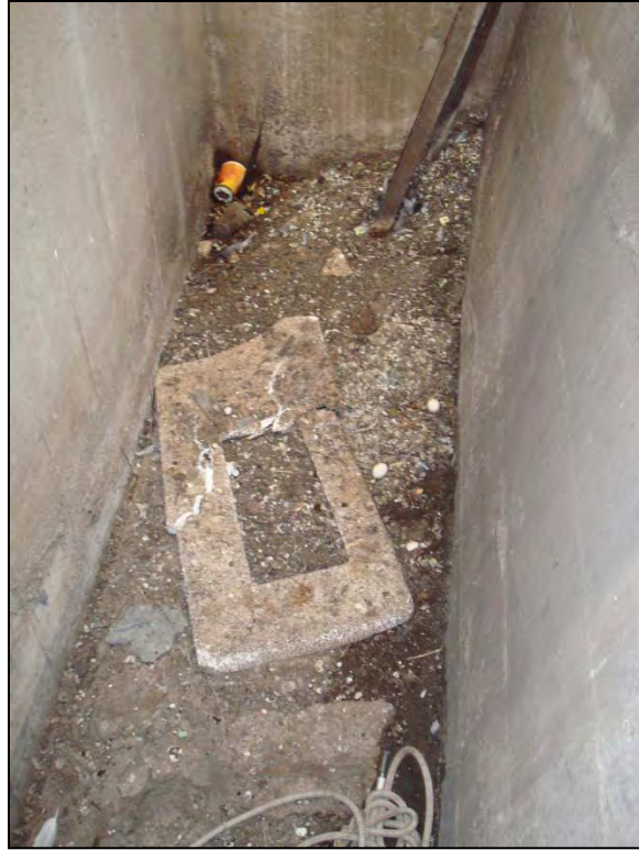
Photo E2-09(ID E111) – Heavy debris (dirt, garbage, bird waste, etc.) at base of arch floor at west face of Pier 2
