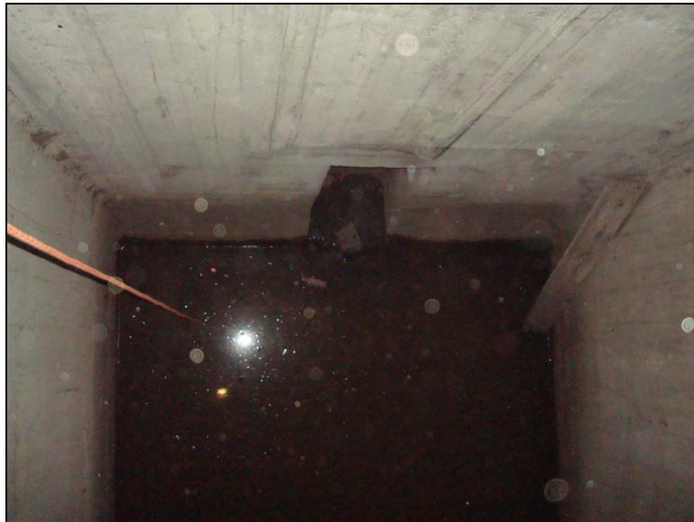
Photo E3-29 (ID E336) – Looking down at lower chamber in Pier 2, access door on east face. Trapped water and debris in base of pier.
