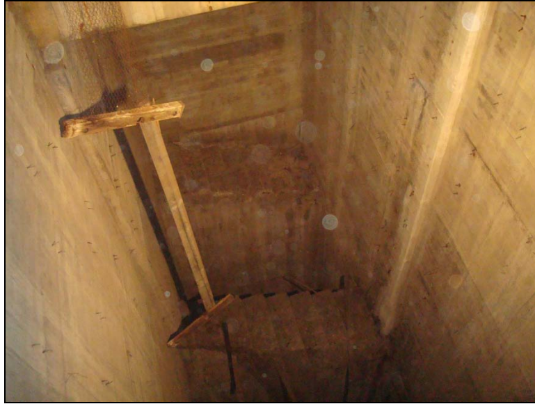
Photo E3-25 (ID E327) – Typical condition, interior of Pier 2. No significant deficiencies noted.
