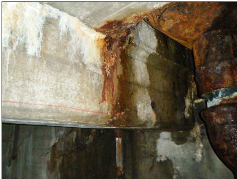
Photo D1-10 (ID E008) – West end of Beam 1 inside Pier 2, note heavy leakage through scupper pan, extensive rust staining, and efflorescence on concrete beam.
