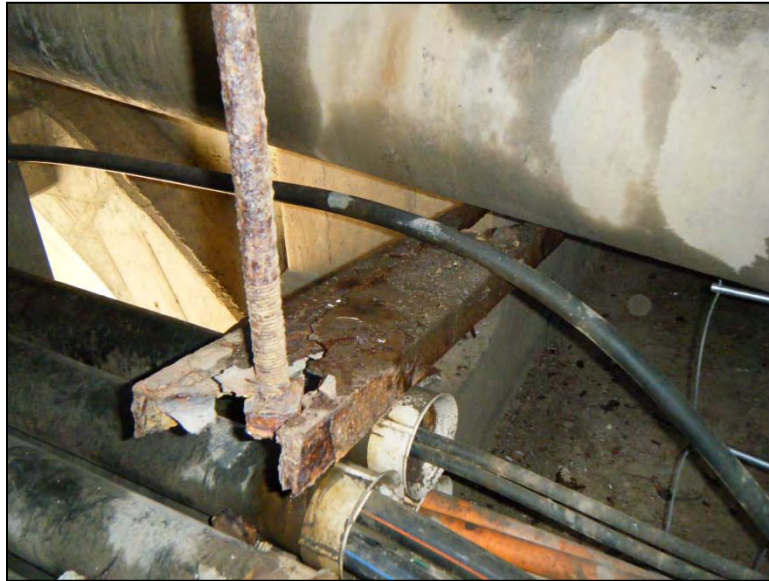
Photo D1-27 (ID E019) – Failed steel utility support bracket near east wall of Pier 2. Bracket supports a 12” dia. pipe.
