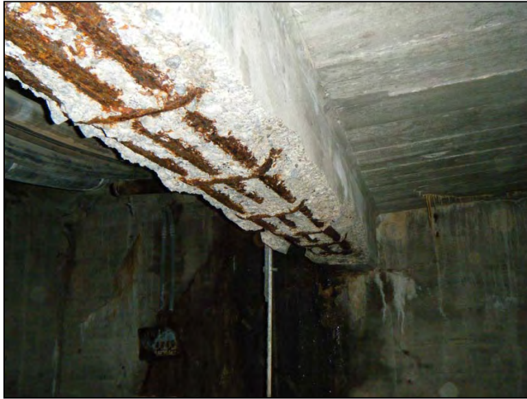
Photo D1-20 (ID E013) – Full length spall on bottom face of Beam 10 in Pier 2. 1/8" section loss to bottom bars and stirrups.
