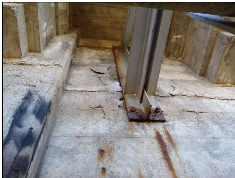
Photo C3-43 (ID C233) – Span 3, Spandrel Wall D between Floorbeams 8 & 9. Multiple localized delaminated areas and spalls, some with exposed reinforcing steel. Bars exhibit up to 1/16" section loss. Also note corrosion on steel utility bracket.
