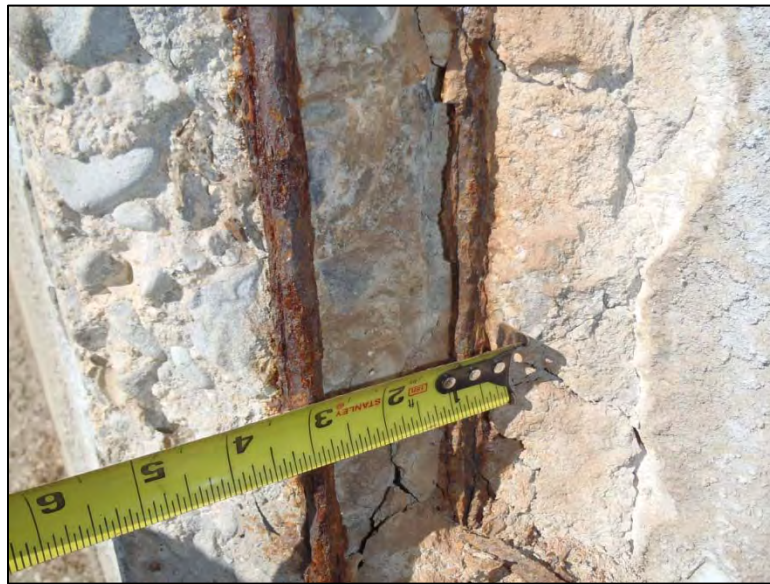
Photo C2-45 (ID C136) – Span 3, Spandrel Arch A, below Floorbeam 8. 5' tall spall along corner, 2 layers of bars exposed. Max loss to bar diameters = 100%.
