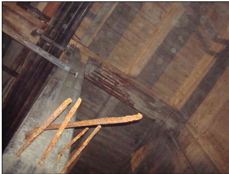
Photo C4-48 (ID M401) – Spalling and bars with section loss (estimated at 1/8" max loss to diameter) on bottom of floorbeam at Column Line 1 in West Approach.
