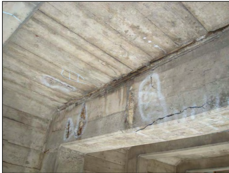
Photo C4-42 (ID C330) – Span 3, Floorbeam 4 at midspan between Spandrel Arches A & B, 4' long x full width x 3" deep delaminated area with spalling. Multiple spalls and delaminations at midspan also noted. Exposed bars in photo have up to 1/8" loss in diameter.
