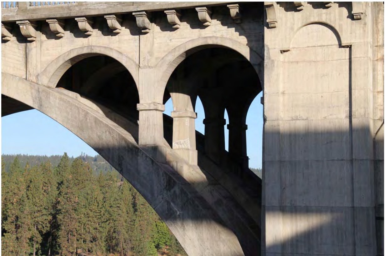
Photograph 2 - Spandrel Columns and Intermediate Arches
