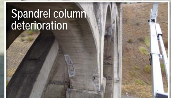
Spandrel column deterioration
