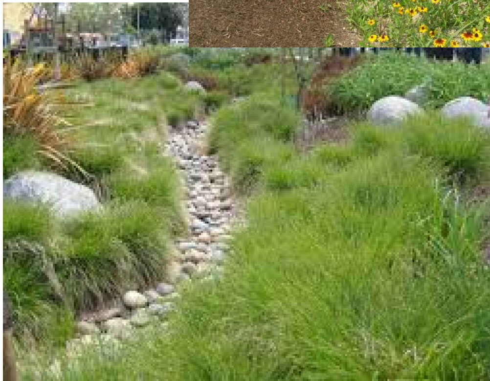
BIORETENTION STORMWATER SWALE CHARACTER
