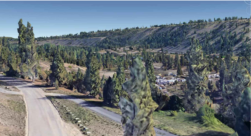
SOUTHWEST SITE FRONTAGE FROM MARSHALL ROAD
