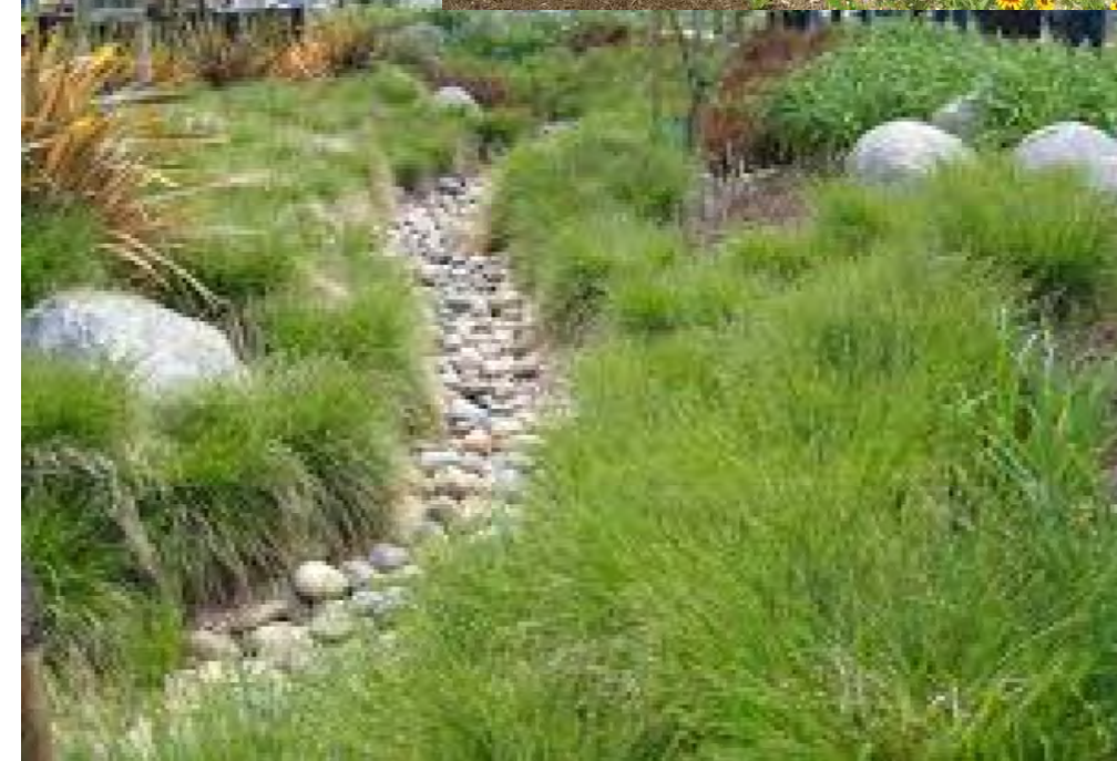
BIORETENTION STORMWATER SWALE CHARACTER
