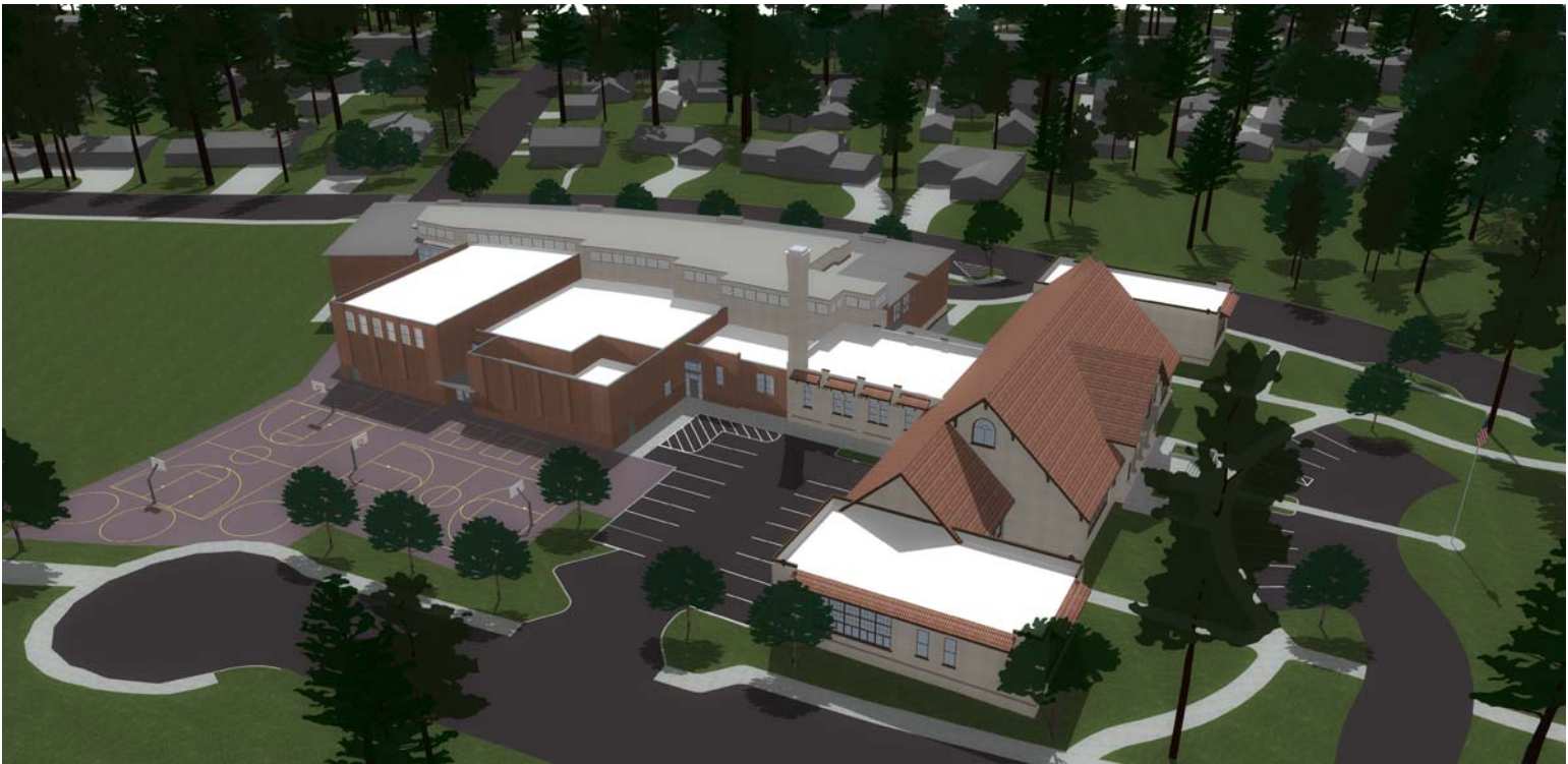
VIEW FROM NORTH
