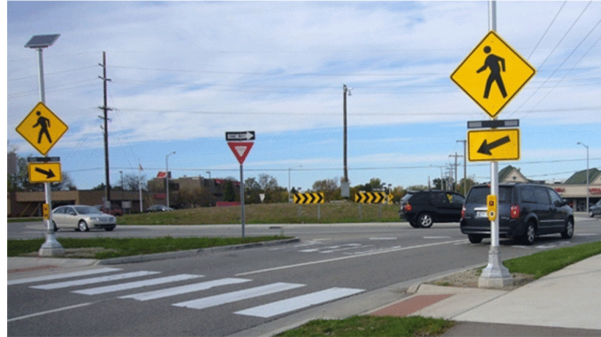
Rapid Rectangular Flashing Beacon (RRFB) at multilane roundabout in Oakland County, MI.
