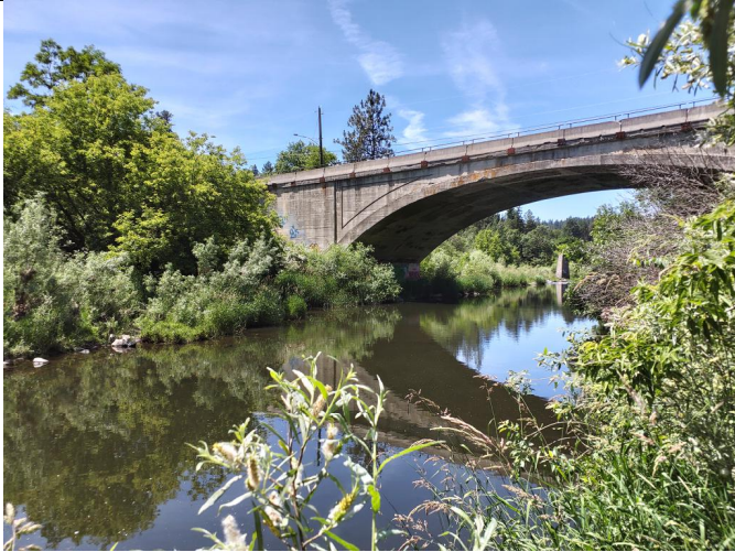
Photo 9: Options 1a and 1b, Latah Creek and Marne Bridge.
