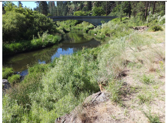
Photo 6: Option 2, Latah Creek and 11 th St Bridge.
