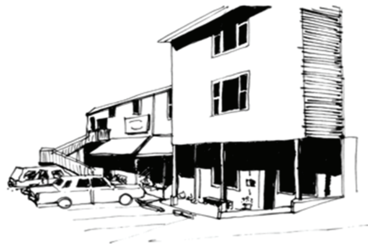
Backside of the building viewed from adjacent residential road
