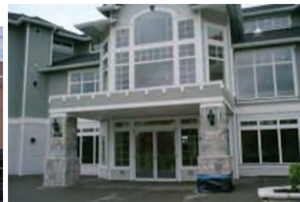
Entrance with portico and ornamental treatments
