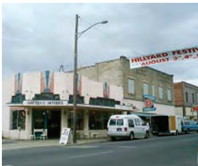
Building with no setback from sidewalk
