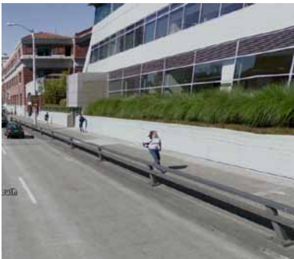
Example of a low rail adjacent to 5 lanes of fast moving traffic in Seattle.
