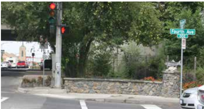
Basalt wall, column and sculpture at 4th and Division Street. Stone sizes range from 2" x 4" depth to 8" x 4" depth, gray mortar.
