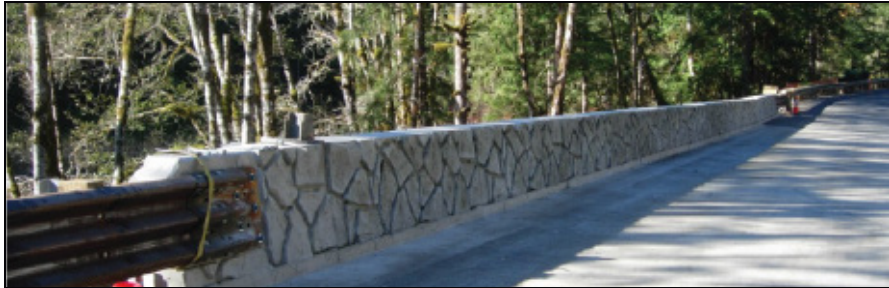
Aesthetic Traffic Barrier - Cast in Place Stamped and Stained Concrete. (Photo taken on SR 542 Church Mt. Rd.)
