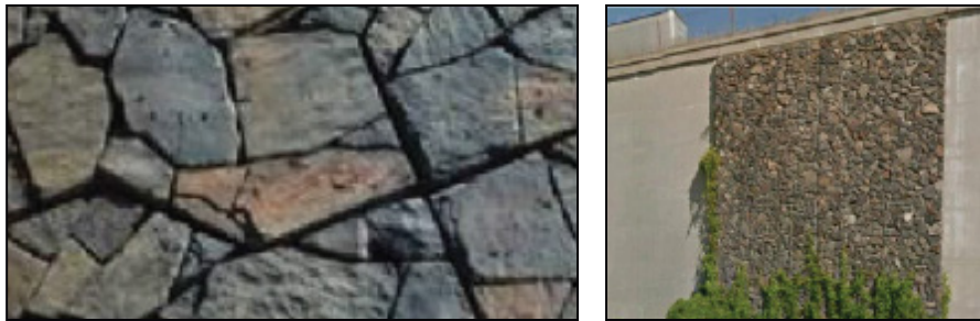
Above Left - Simulated basalt - integral color, stamp and stain. Above Right - Color and pattern of basalt veneer walls on I-90 main line to be used as a model for aesthetic traffic barriers.
