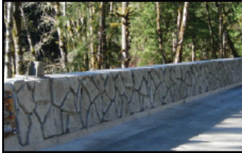
B - Aesthetic Traffic Barrier - Cast in Place Stamped and Stained Concrete.
