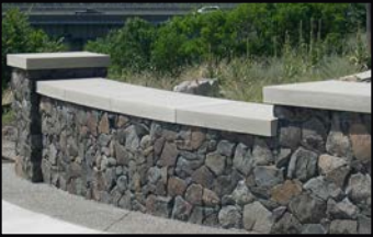
A - Genuine Basalt Wall with Cap (photo taken at Kendall Yards).
